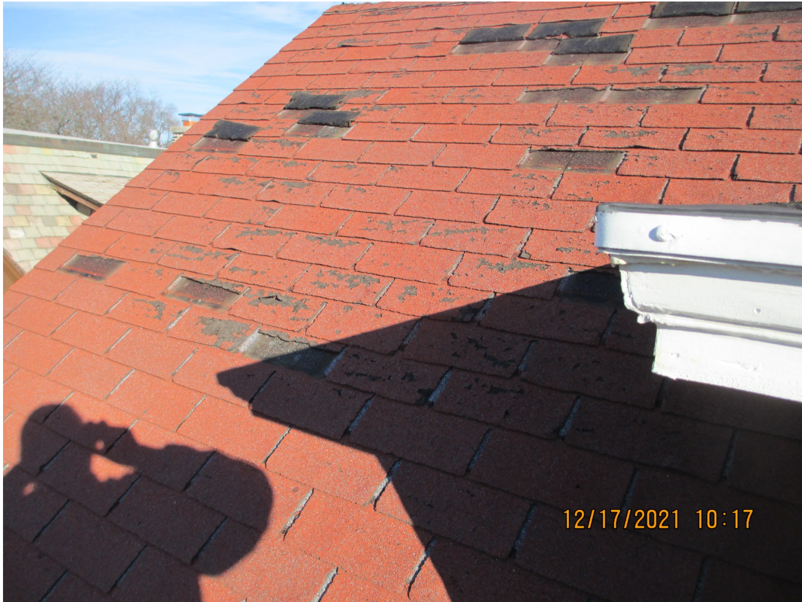
Existing roof condition
