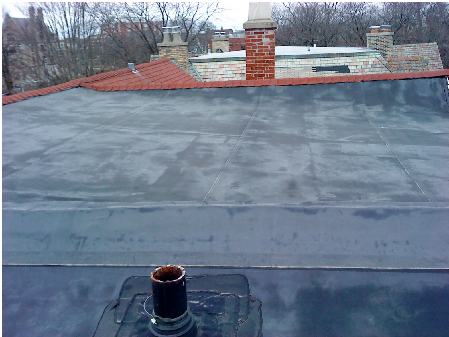
Existing roof condition
