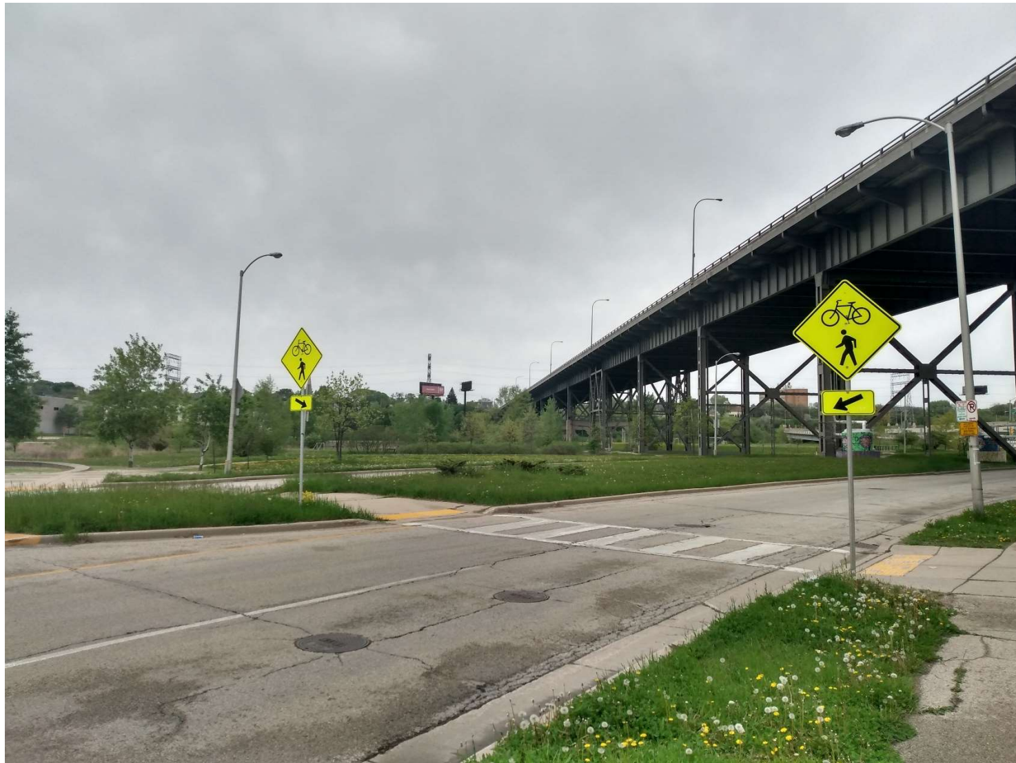
Picture C: The HAST crossing in the Menomonee Valley, looking northwest. Here, the signs alert drivers to both pedestrians and cyclists.
