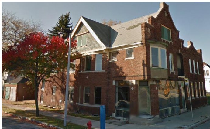
East Side of Building
