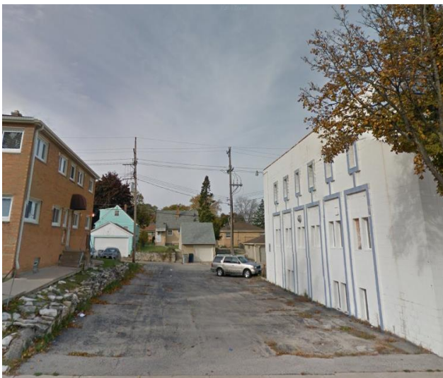
Parking along south side of building.
