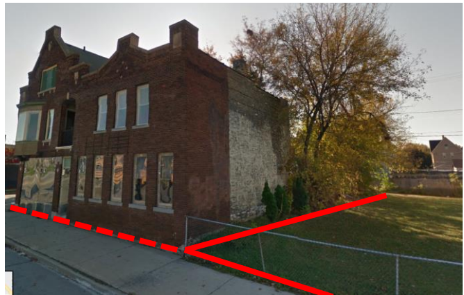
West Side of Building and Lot
