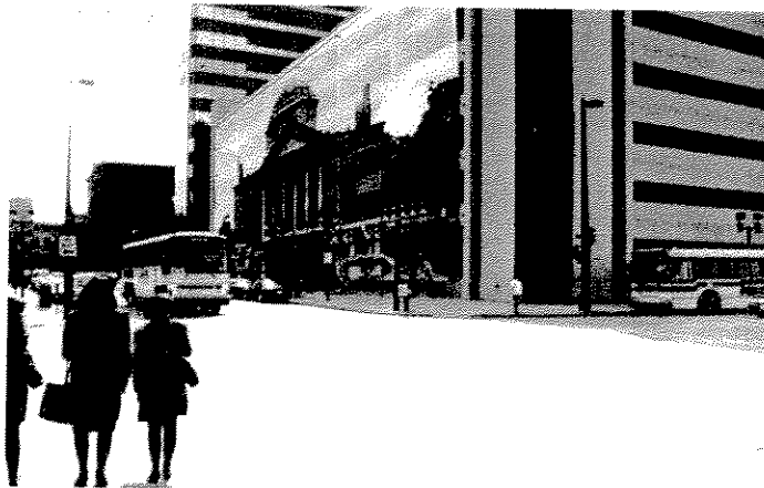
Proposed Parking Deck Screen has a printed image, a technique popular in Europe. This is an inexpensive way to enhance the streetscape image of existing decks.
