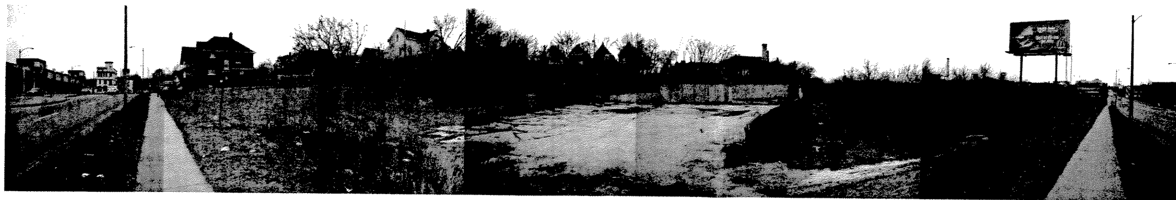
PANORAMIC VIEW OF SITE, LOOKING WEST, NORTH AND EAST
