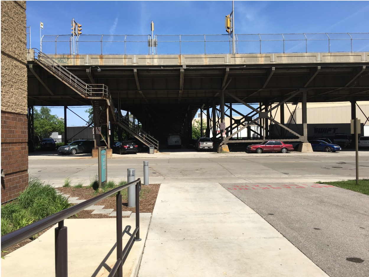
Looking east, across W. Potawatomi Circle, from the location of the proposed infill building.
