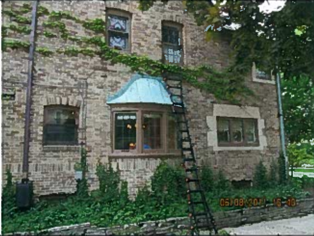
North side repairs to prevent leaking
