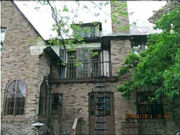
Flat roof at rear of house to be removed and replaced with copper. May have iron/steel railing installed
