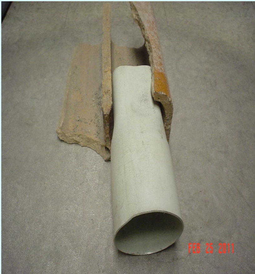
PVC Pipe in Clay Duct
