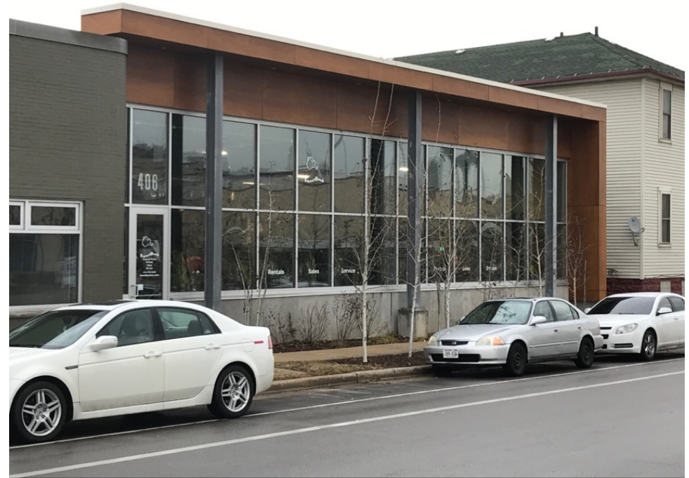
New construction in 2017, 406 West Walnut
