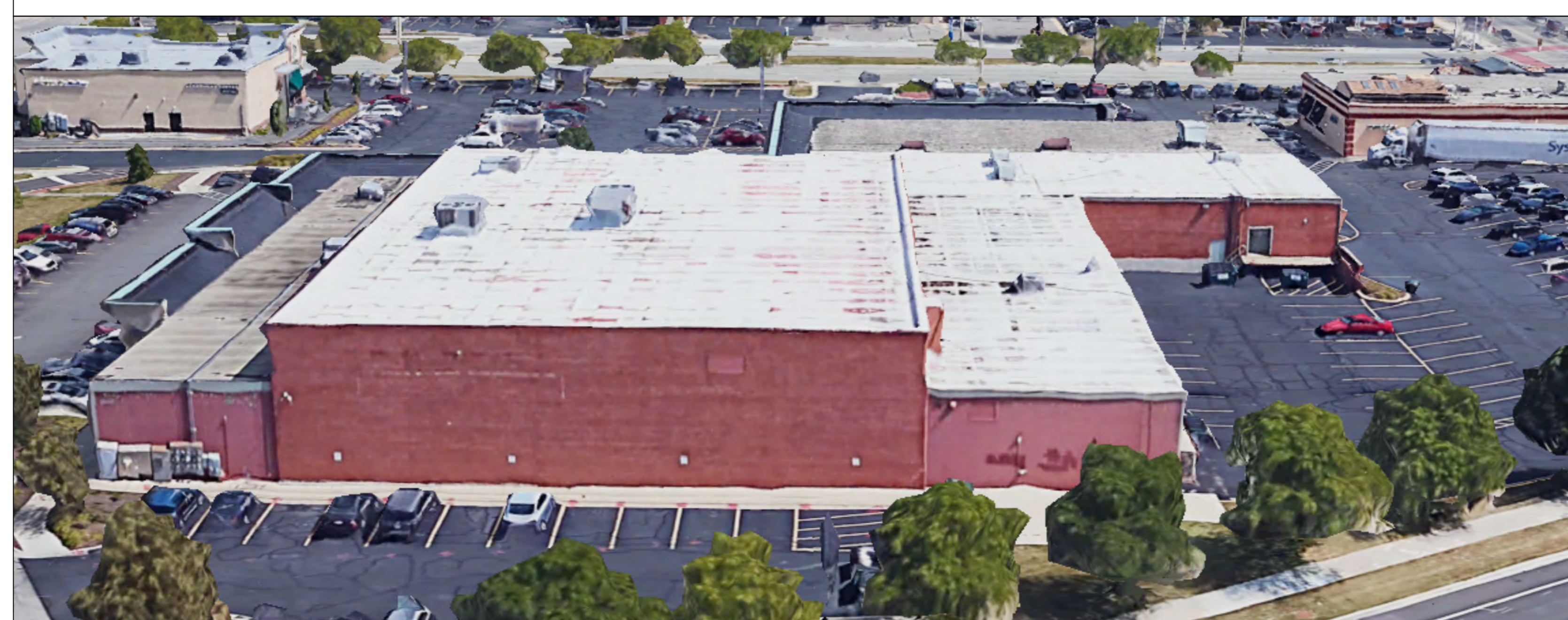
EXISTING WEST ELEVATION LOOKING EAST
