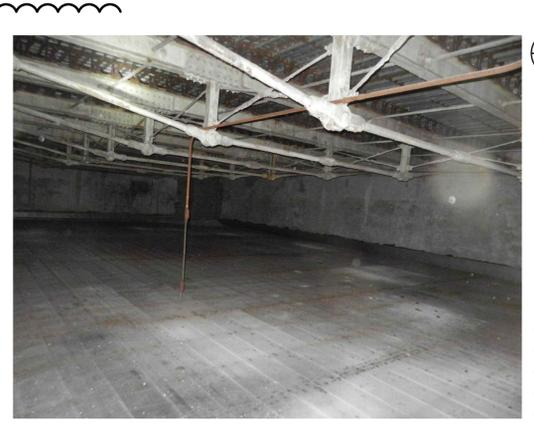
(M1) EXISTING STEEL TRUSSES FROM EXISTING FURNACE AT BUILDING #25 TO BE REPURPOSED IN THE TWO STORY ACTIVITY ROOM AT THE LOWER LEVEL FLOOR.
