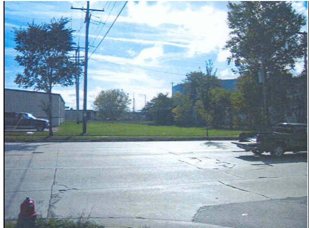
View Looking South
