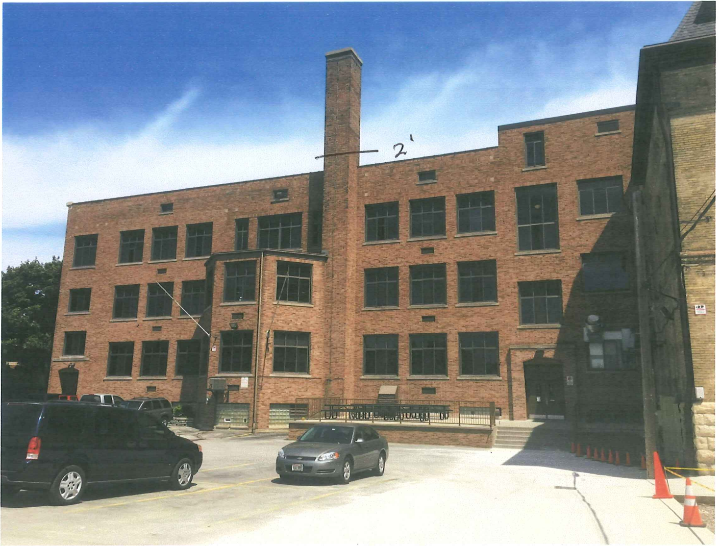
SCHOOL WEST ELEVATION OF CHIMNEY
