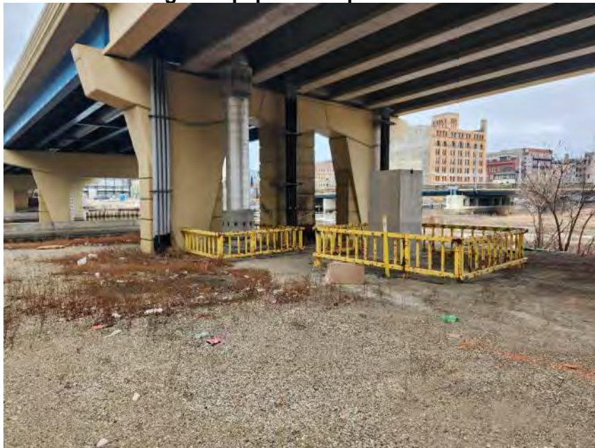
We Energies Equipment to protect with fence
