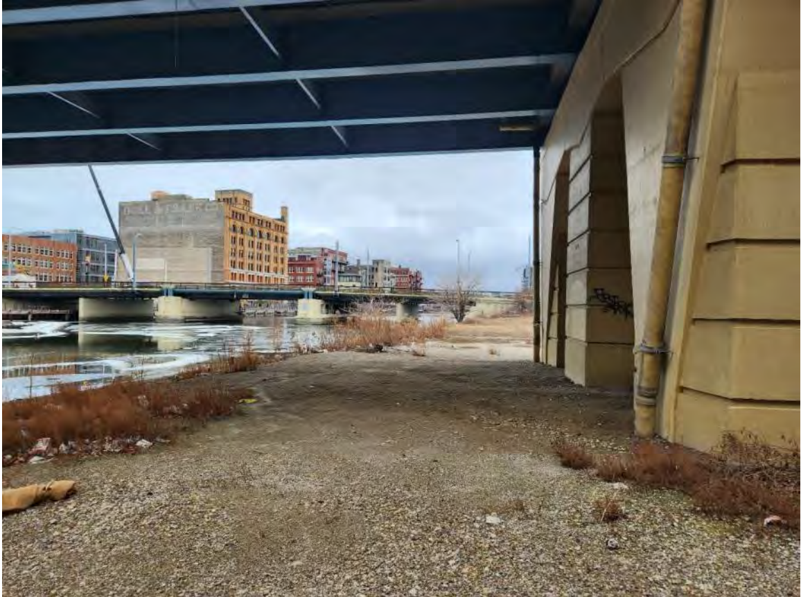
Looking South along Riverwalk area, where trail would be located (between waters edge and east side of Dog Park)
