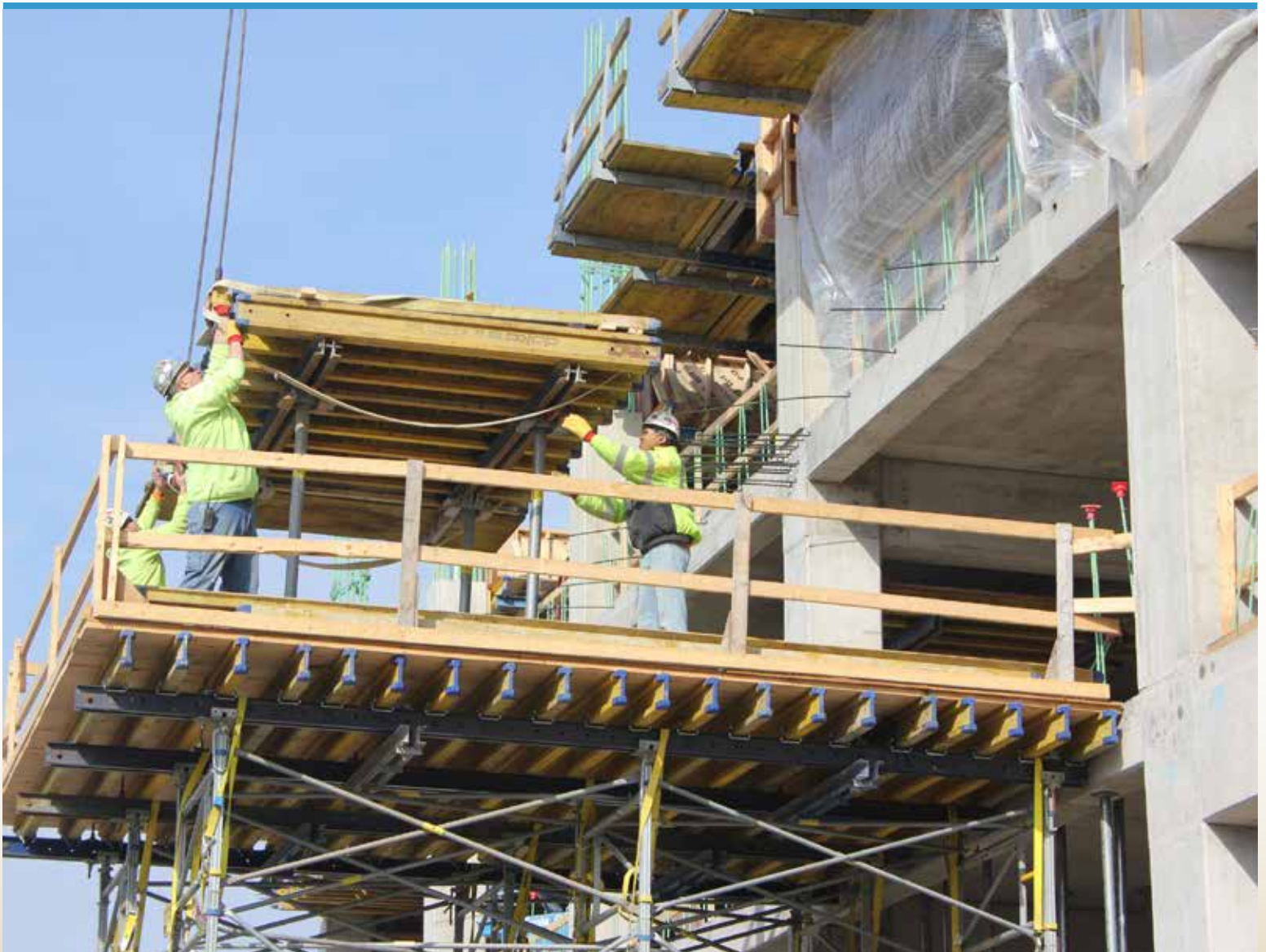
Workers moving materials on the Block 7 Parking Structure site.
