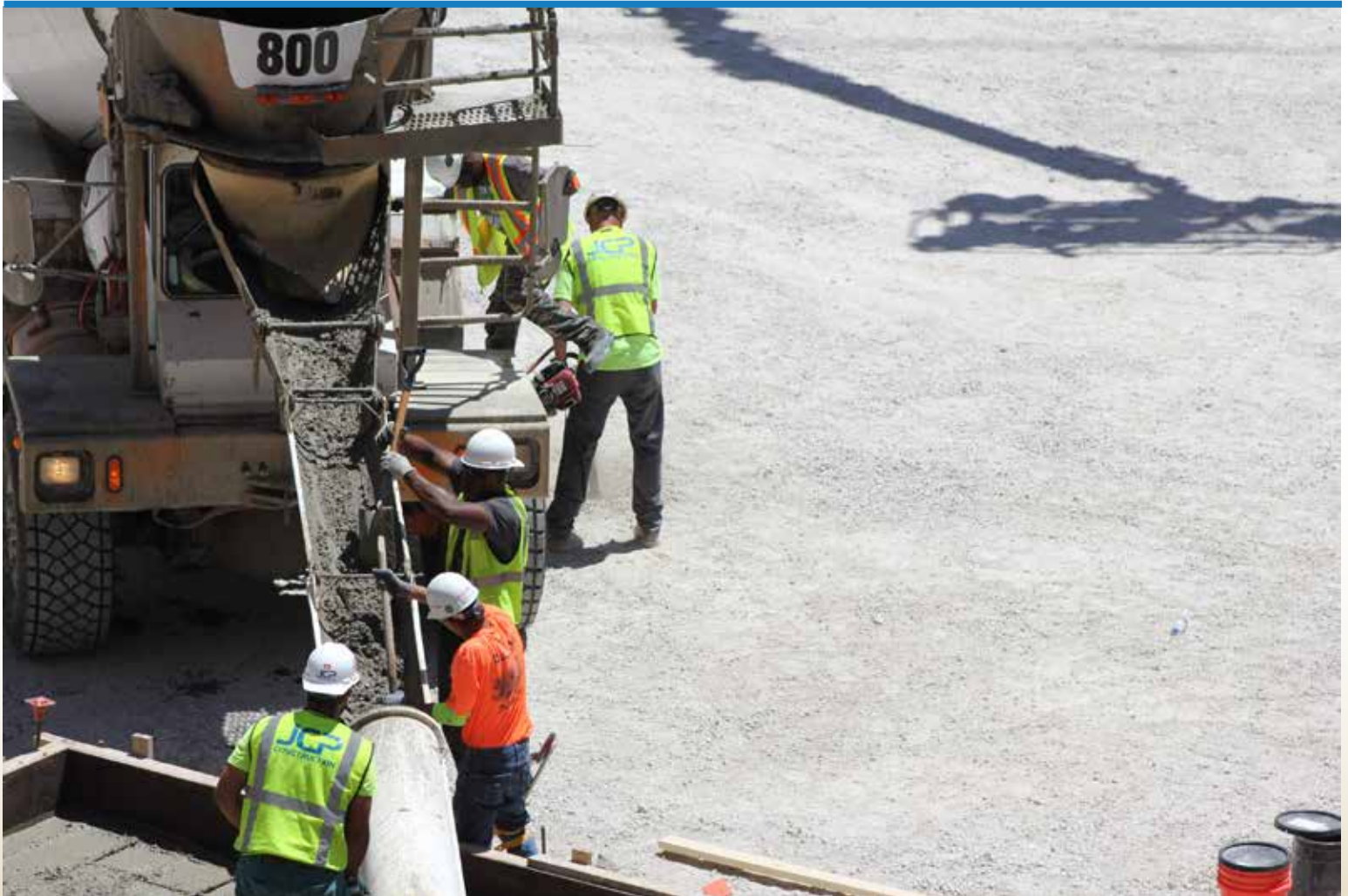
Workers pouring concrete on Arena project site.
