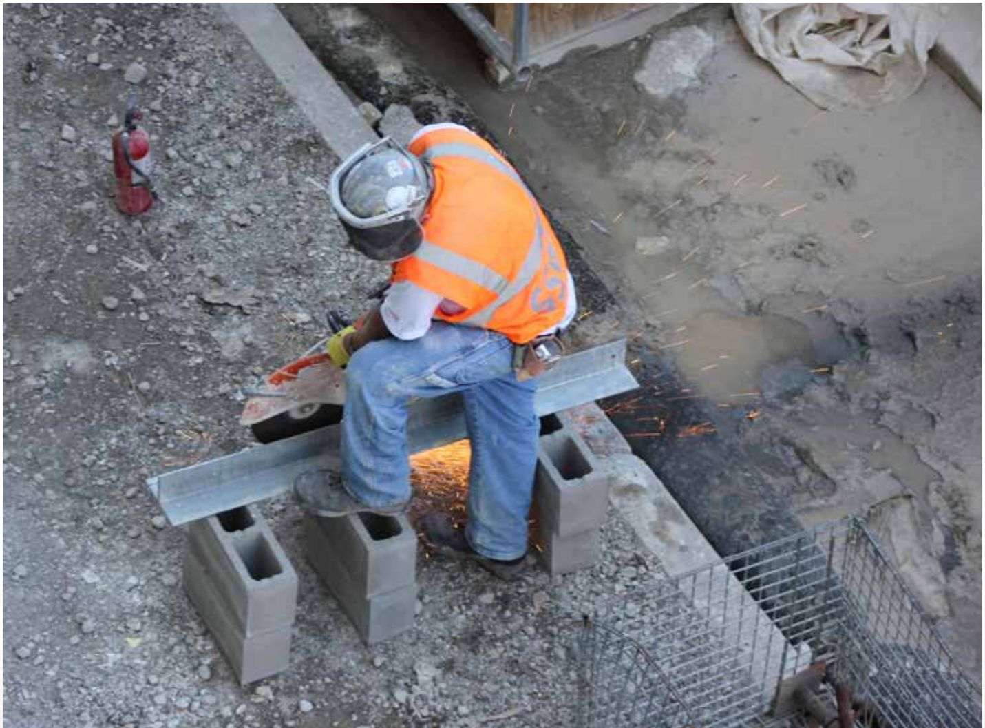
Worker cutting steel for the New Milwaukee Arena.
