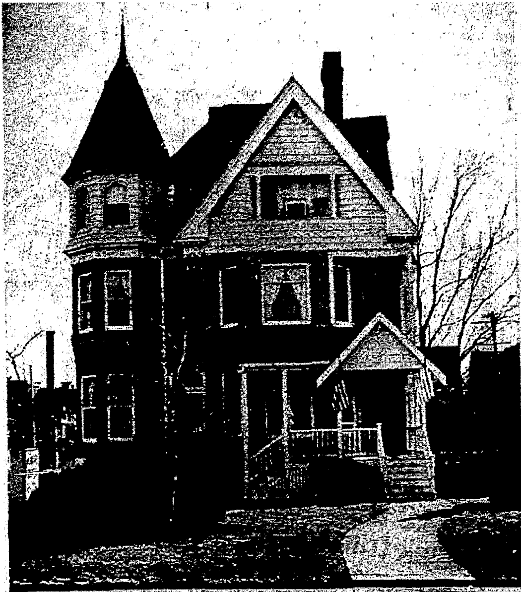
The exterior of the Realtors' building, a home built in 1892, has been restored to its turn of the century appearance. The original porch was duplicated; asphalt siding was replaced by cedar shake shingles on the third floor, the Cream City brick was cleaned and a new roof was added.
