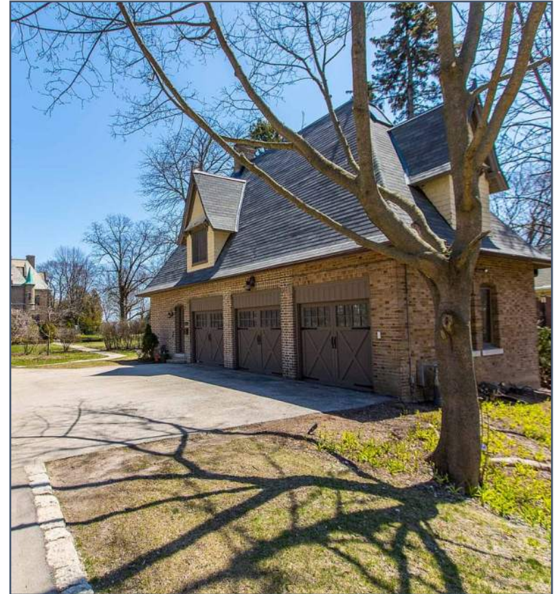
Outbuildings and Structures – Existing Coach House
