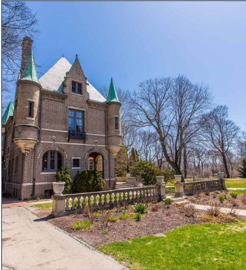
Landscape – Existing Balustrade
