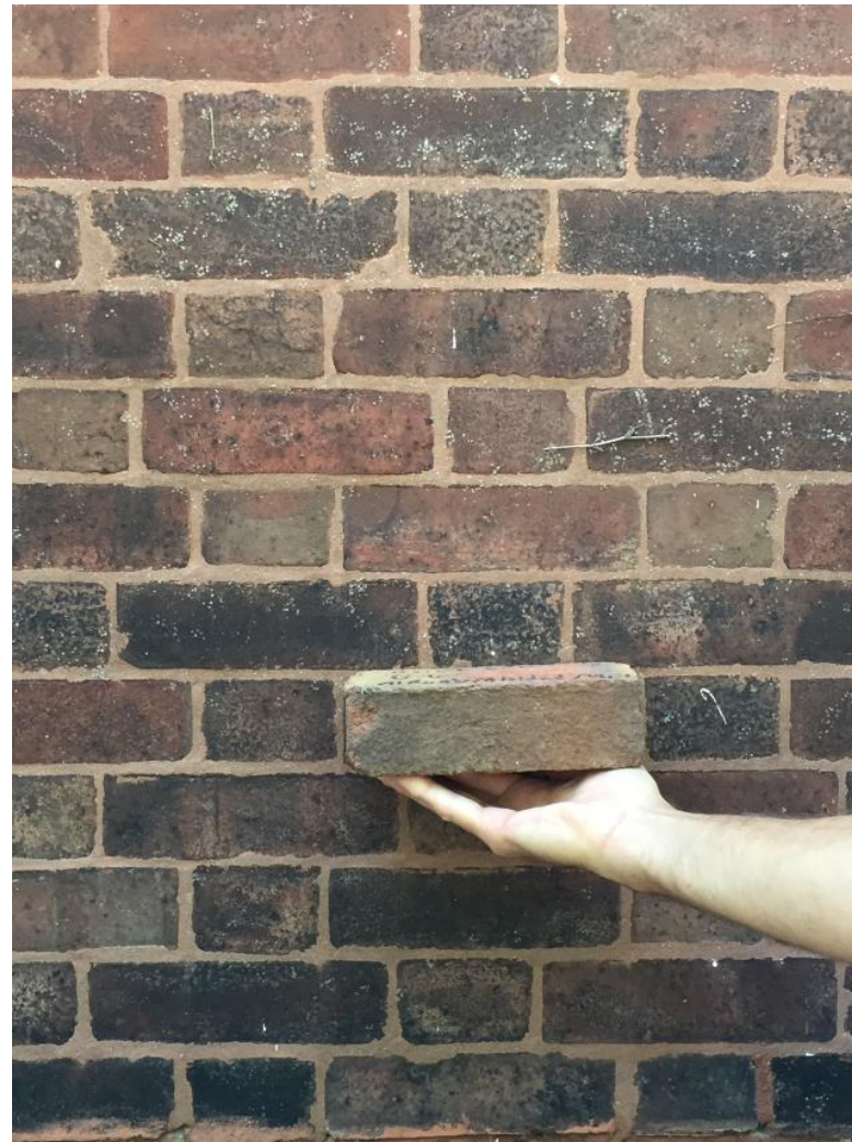
Detail images of (Left) the mortar sample, coursing sample (indicating Flemish bond) and (Right) brick to be utilized for infill at this location and for the reconstruction of the southern chimney
