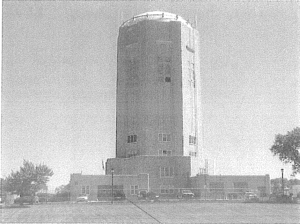
Fig 2 EXISTING Elevation Looking East
