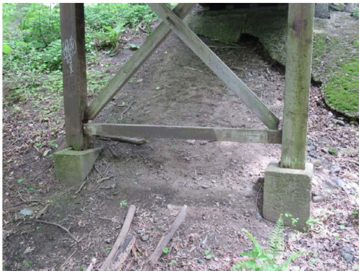
Photo E. Wood Columns/Concrete Piers.
