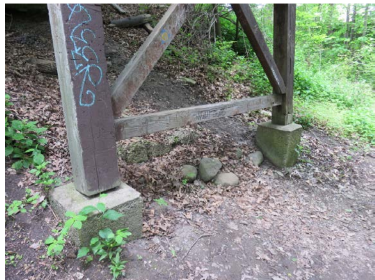
Photo F. Wood Columns/Concrete Piers.
