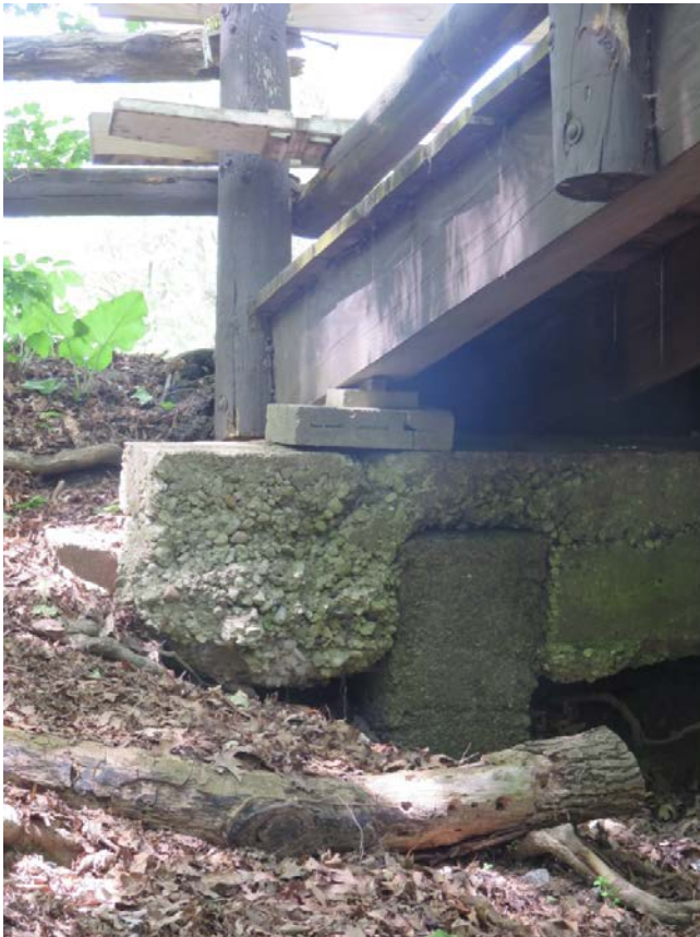
Photo C. North Concrete Foundation.
