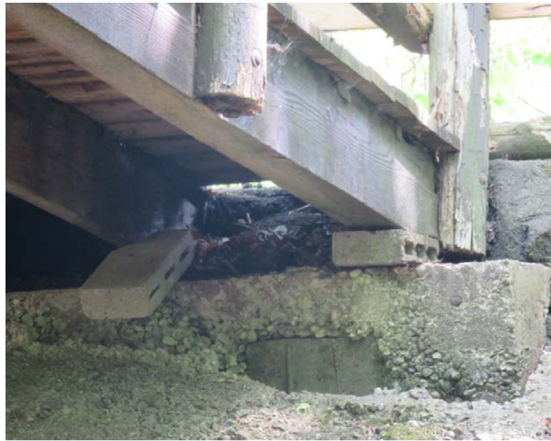
Photo D. South Concrete Foundation.
