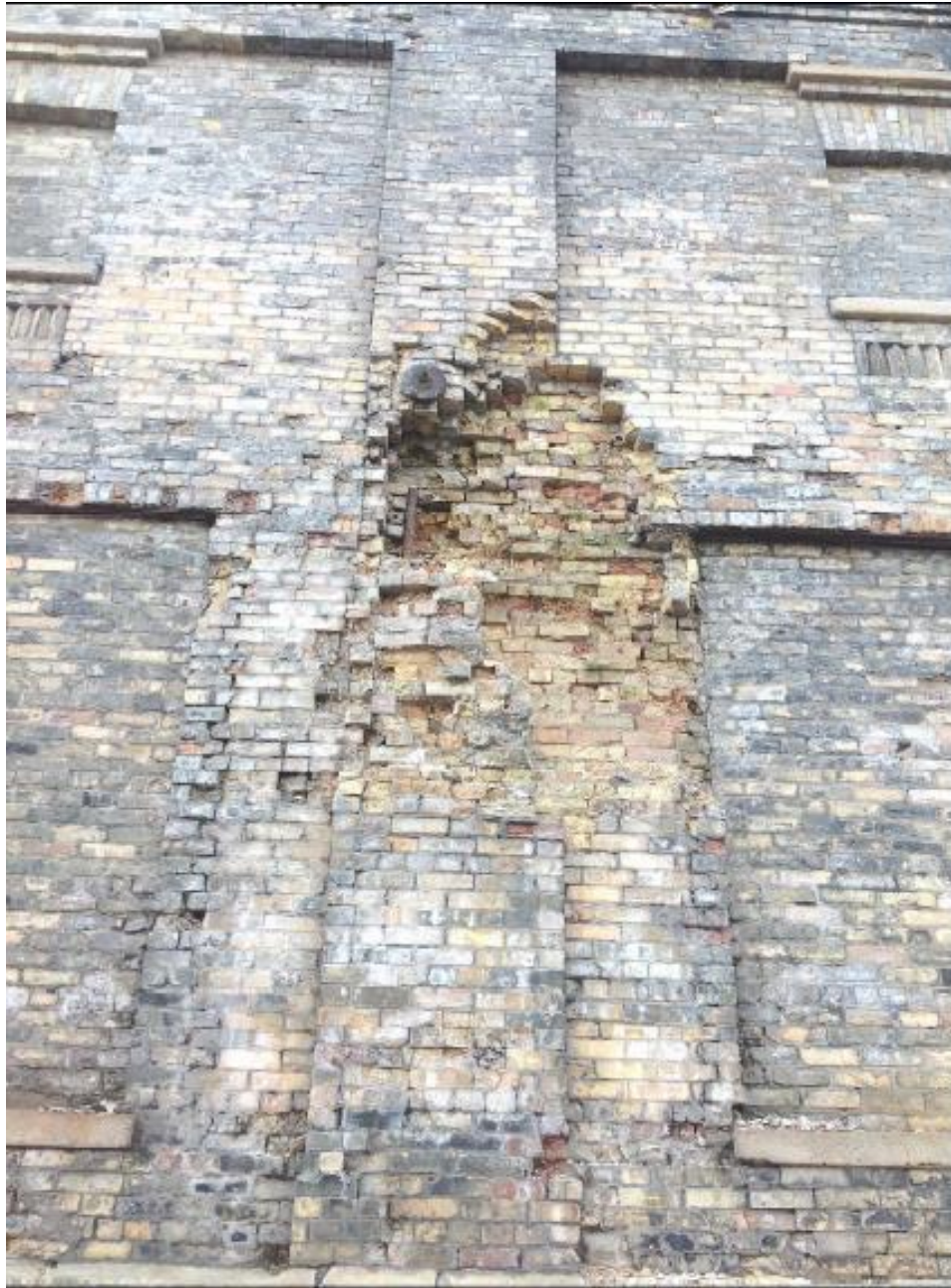
Photo 10: Masonry deterioration on north elevation of Building 25.
