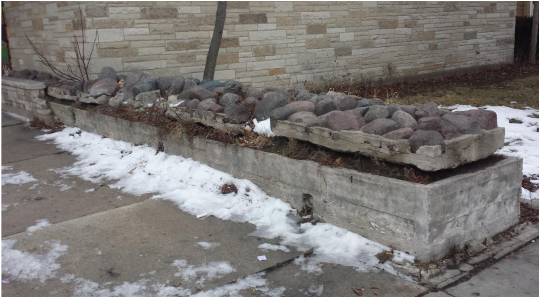
Previous condition of the planter prior to rehabilitation
