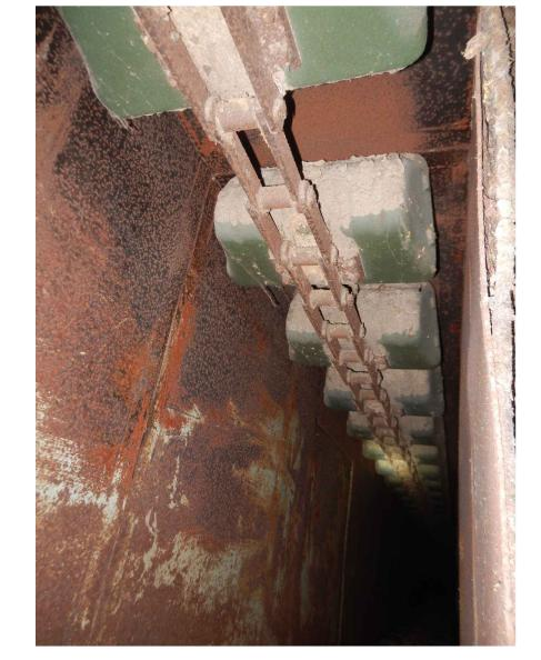
INTERIOR DETAIL OF THE GRAIN ELEVATOR SHOWING THE CONTAINERS AND CONVEYOR SYSTEM TO BE DISPLAYED THRU THE EXISTING HATCH DOORS.
