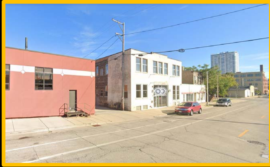
View from N. Vel R. Phillips looking south-east
