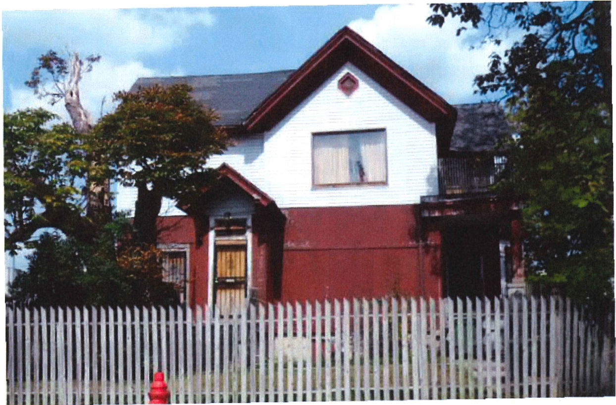
1234-36 West Garfield Avenue
