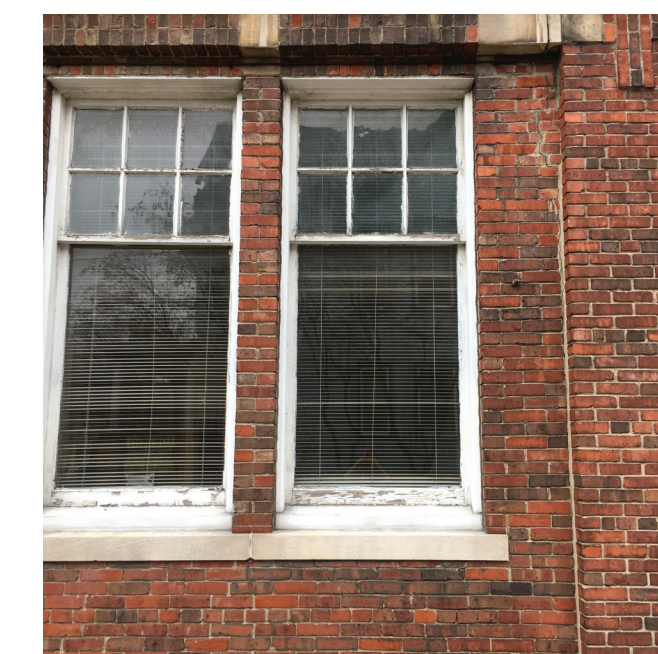
EXISTING MASONRY & WINDOWS
