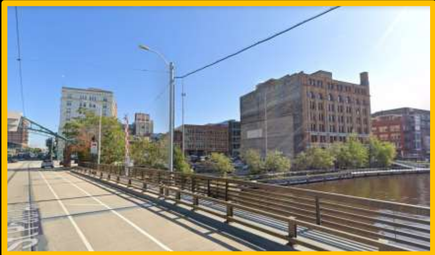
View from East St. Paul Ave looking south-east
