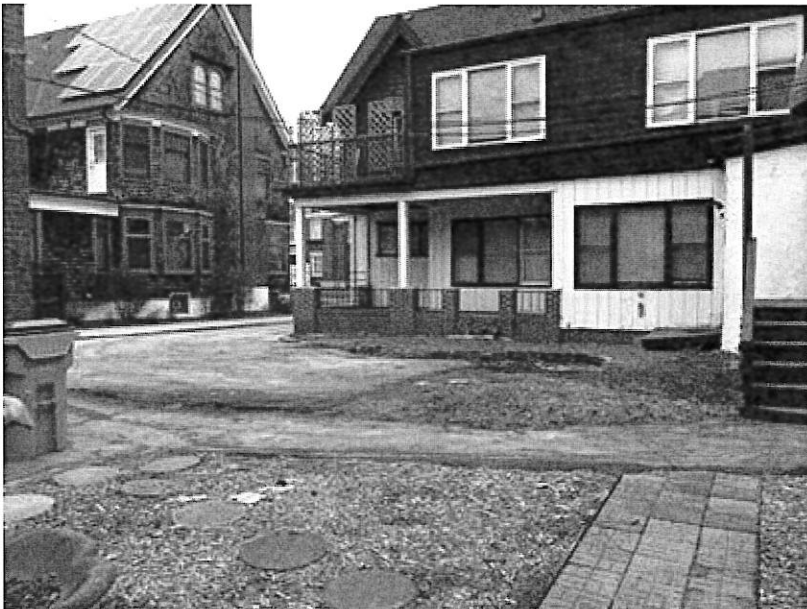
Existing 2727-2729 E Bradford driveway & garage, from Bradford Ave
