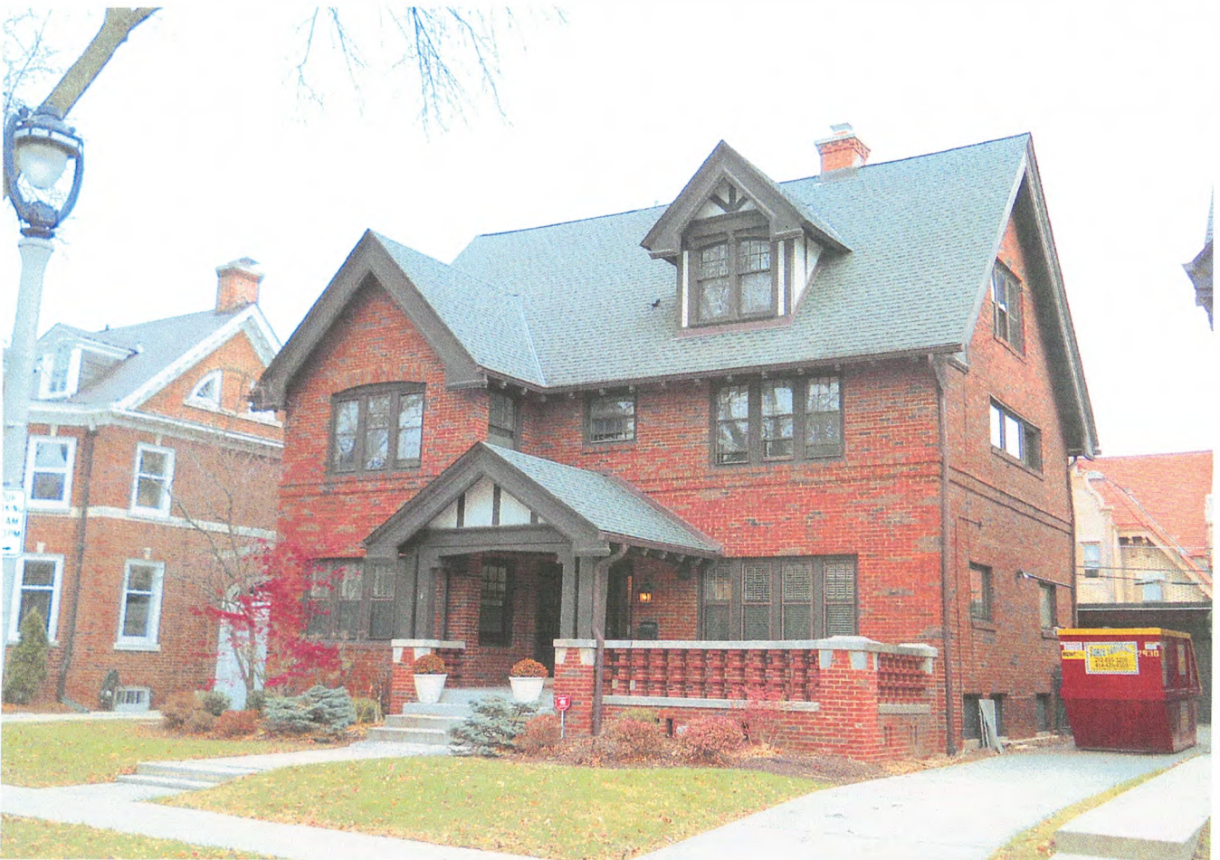
West side of home
