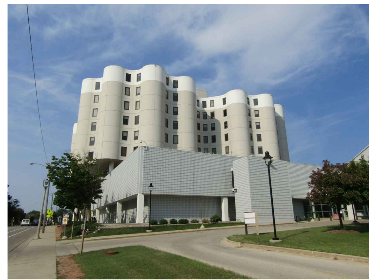
OVERALL VIEW OF NORTH ELEVATION OF WOMEN'S HOSPITAL BUILDING
