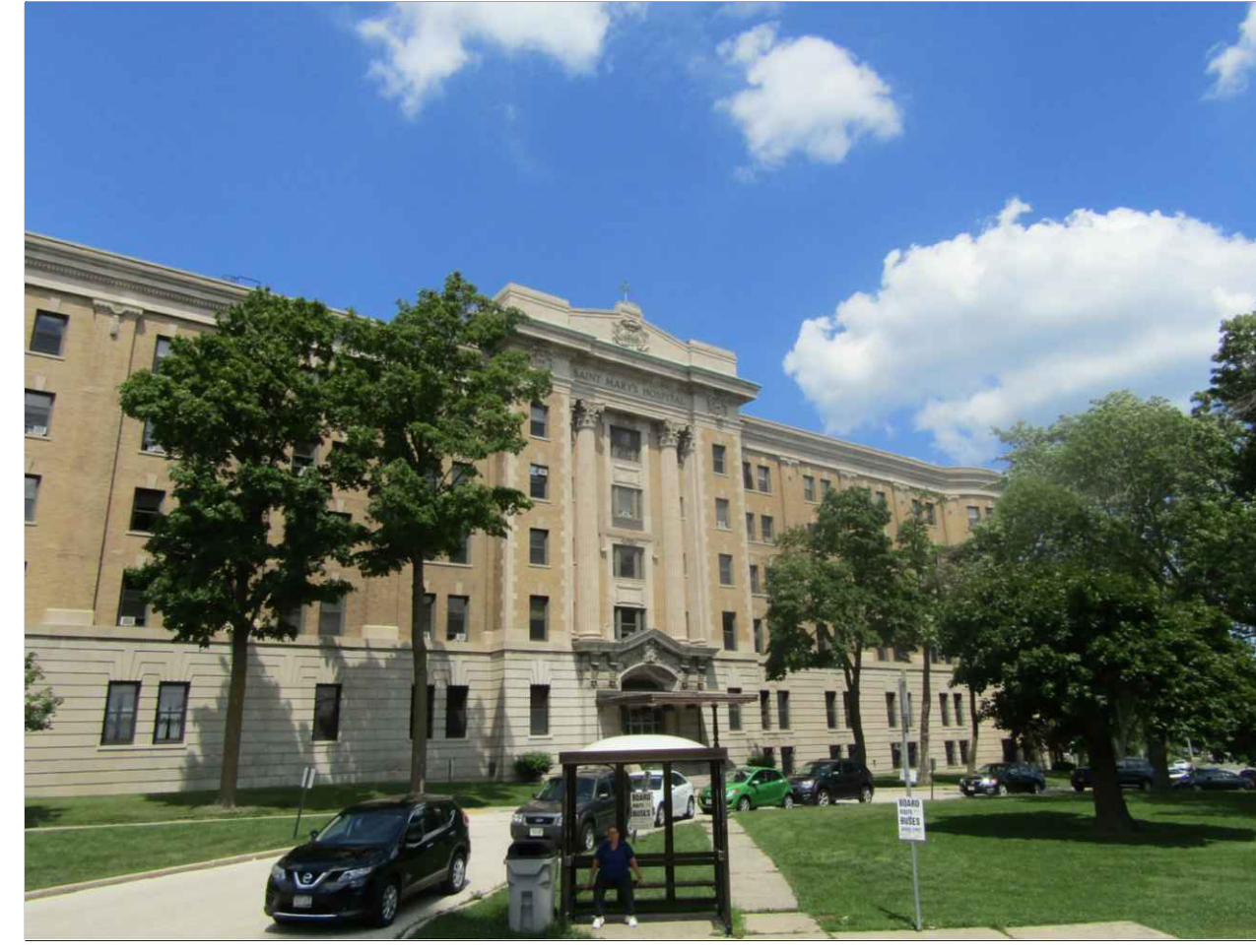
OVERALL VIEW OF SOUTH ELEVATION OF THE HERITAGE CENTER BUILDING
