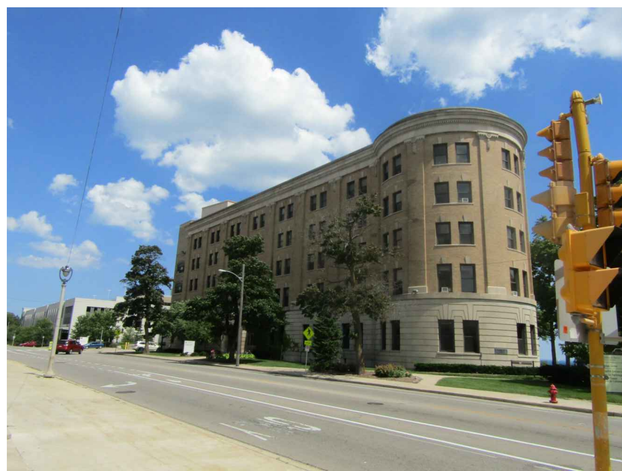
OVERALL VIEW OF WEST ELEVATION OF THE HERITAGE CENTER BUILDING
