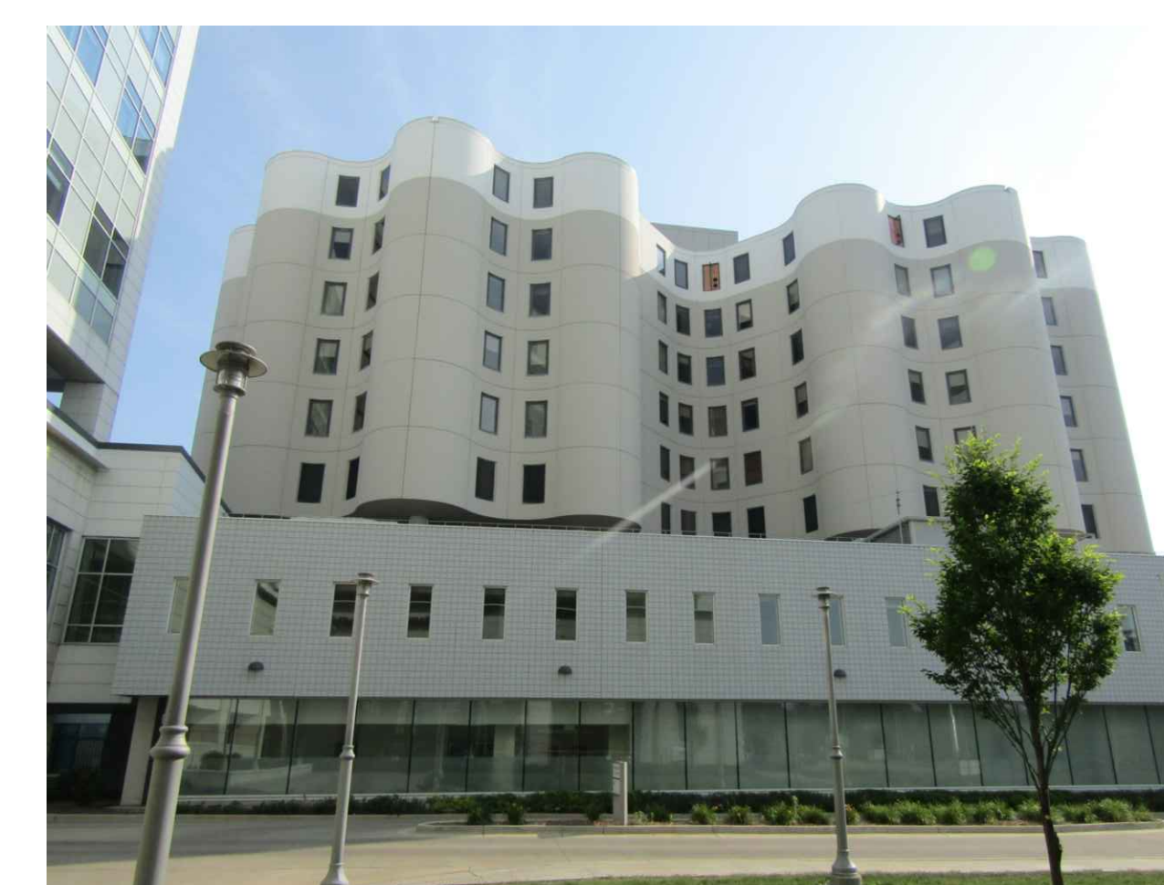
OVERALL VIEW OF SOUTH ELEVATION WOMEN'S HOSPITAL BUILDING
