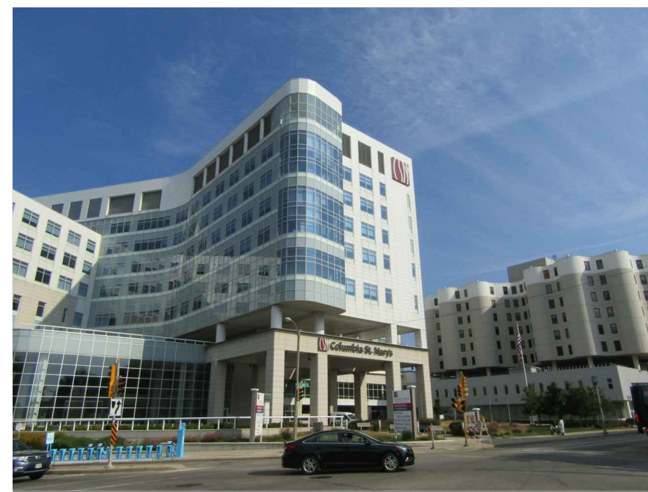
OVERALL VIEW OF SOUTH AND EAST ELEVATIONS OF MAIN HOSPITAL
