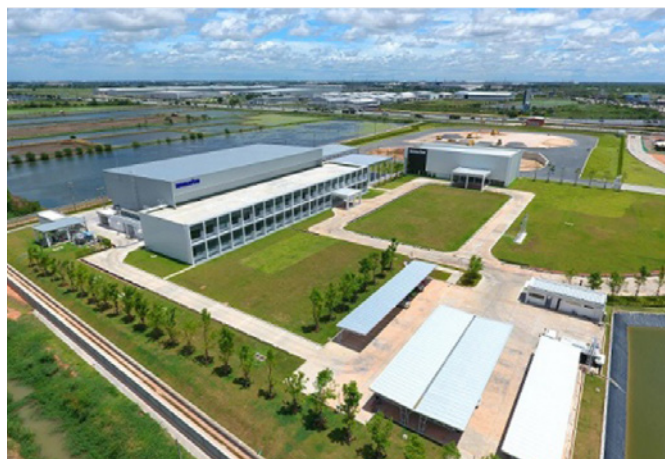
Asia Training & Demonstration Center, built in a suburb of Bangkok, Thailand, began training in November 2016. As part of reinforcing operations in Asia, the Center offers an extensive range of training programs needed for distributors' personnel, including sales of machines and parts, service, and machine operation.
