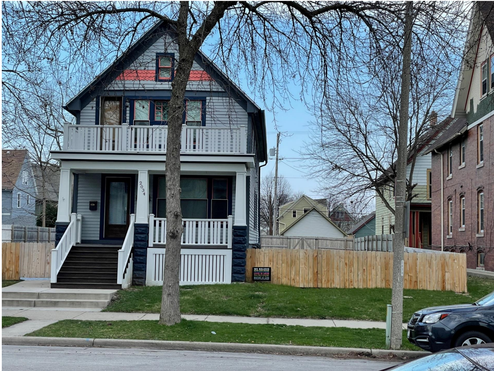
Fence in April 2021. Siting and height are approved if they are zoning compliant.
