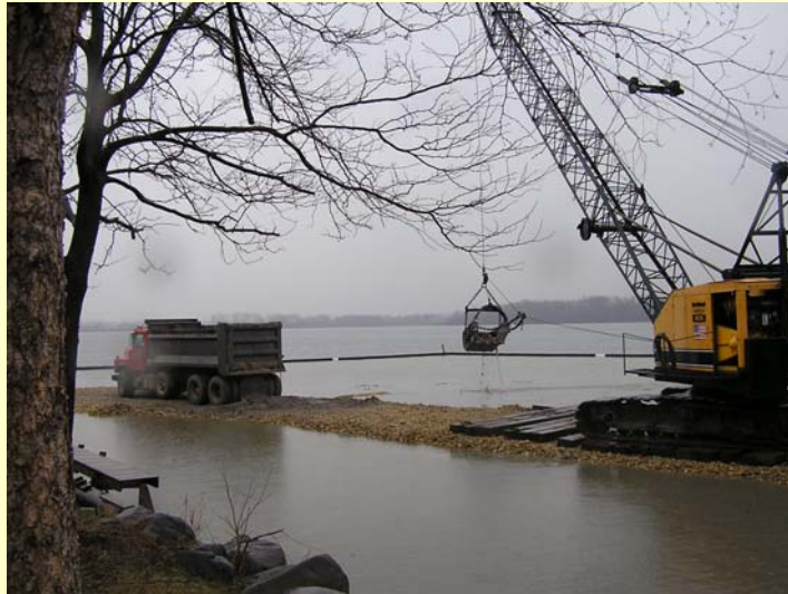
Dredging lakes and streams
