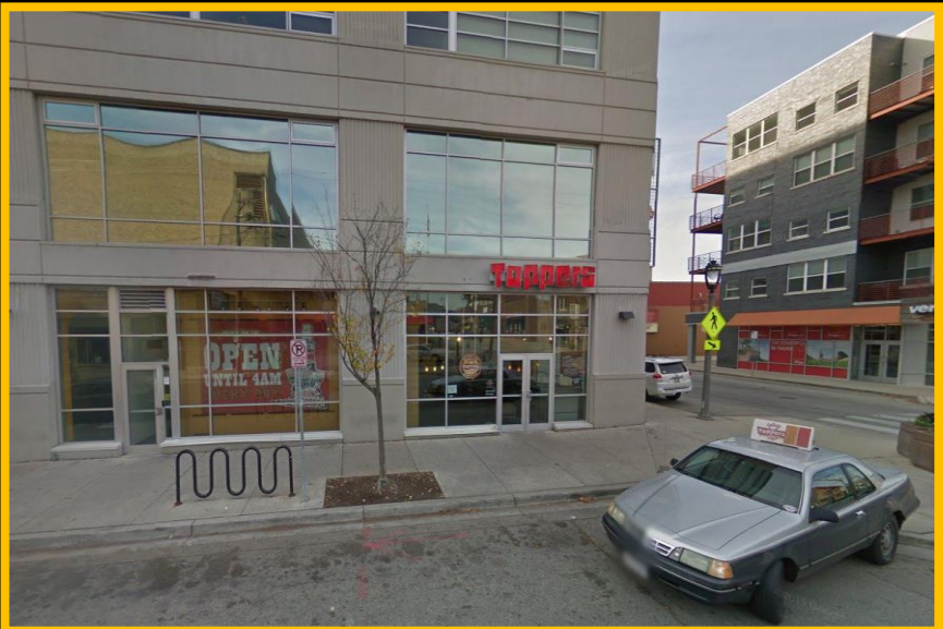
View of North façade from East Kenilworth
