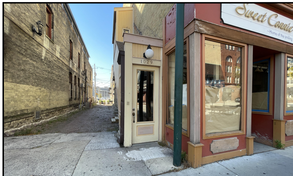
2. STREET LEVEL LOOKING NORTHWEST
