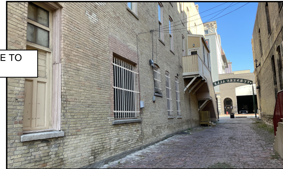
3. STREET LEVEL LOOKING NORTHEAST
