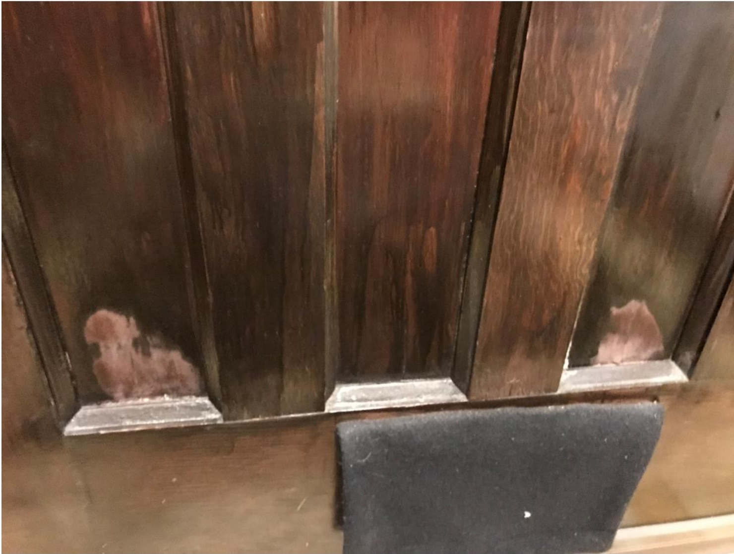
Present condition of the door from the interior
