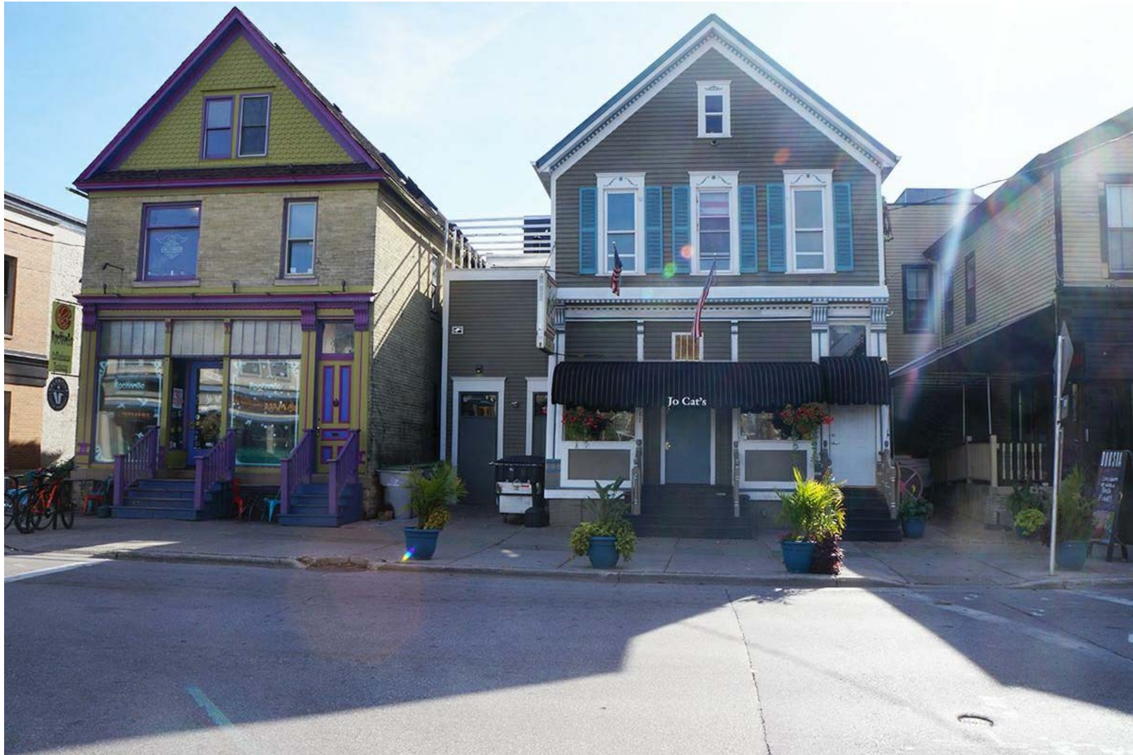
STREET VIEW - FROM NORTH
