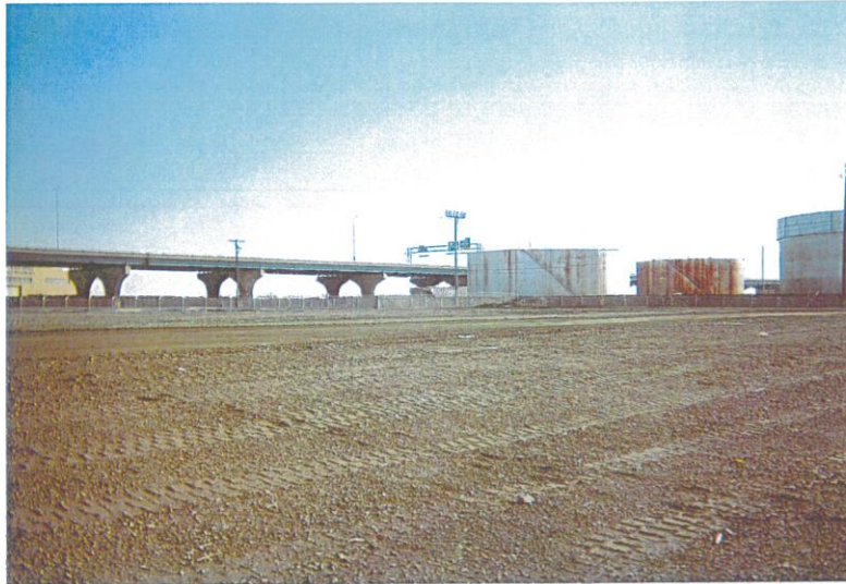
View Looking Southeast Across the Completed Final Cover Over the Former PTW, Inc. Site (12/26/2011)
