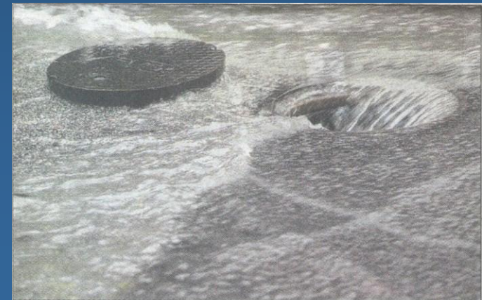
Rushing storm water pushes away sewer covers near E. Locust St. and N. Bartlett Ave.
