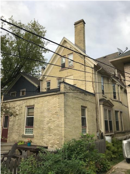
Looking NE towards Rear of House
