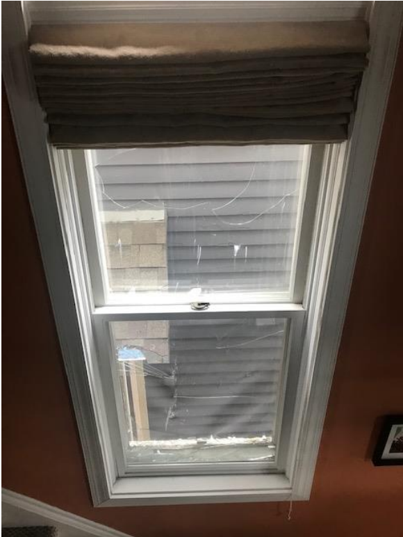
NE Side Window – Interior
