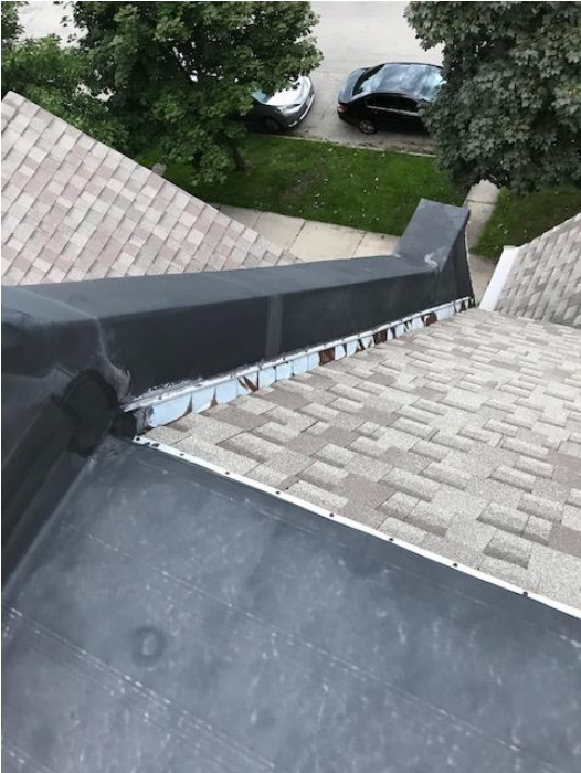
East Side Roof/Parapet Wall
