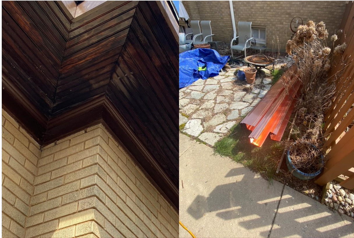
New gutters being installed and sample repaired soffit.
