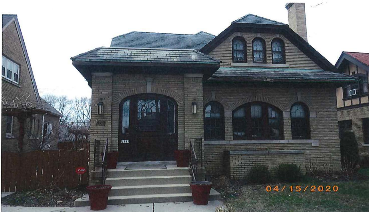
Front of house with work in progress.
