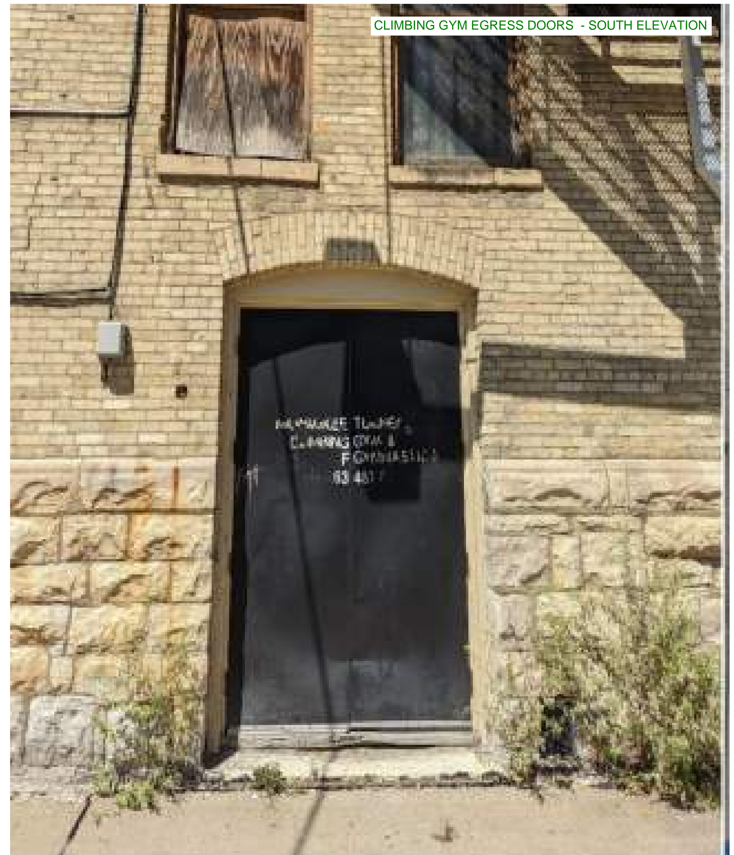
Non-original metal double doors in historic open. Historic opening to remain intact. New single panel metal double doors to be installed in existing opening. Original door configuration unknown.
