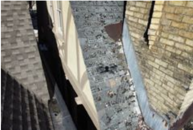
IMAGE 4: South eave at chimney.
