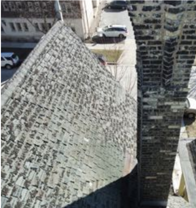
IMAGE 1: South roof slope, east end existing conditions.
