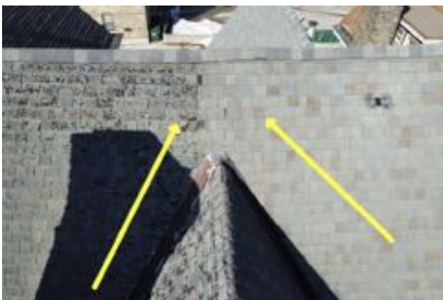
IMAGE 6: East main roof slope where differing roof layers are clearly evident.
