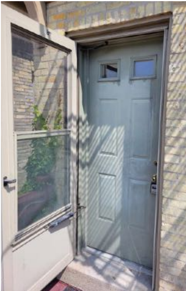
IMAGE 10: Current second floor west (rear) door.
