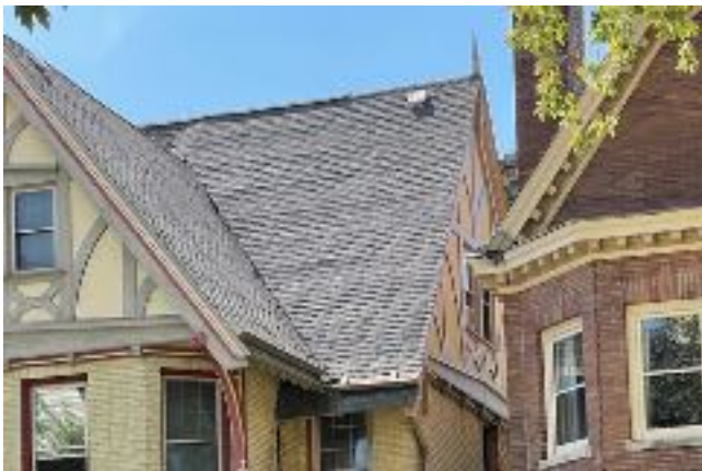
IMAGE 5: North and east roof slopes at the north roof half.
