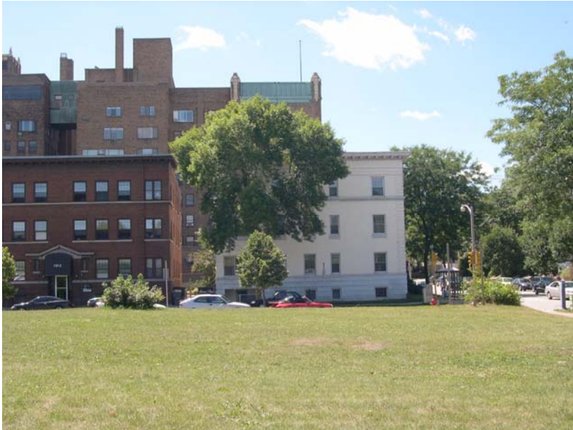
From center of site, towards Lafayette
