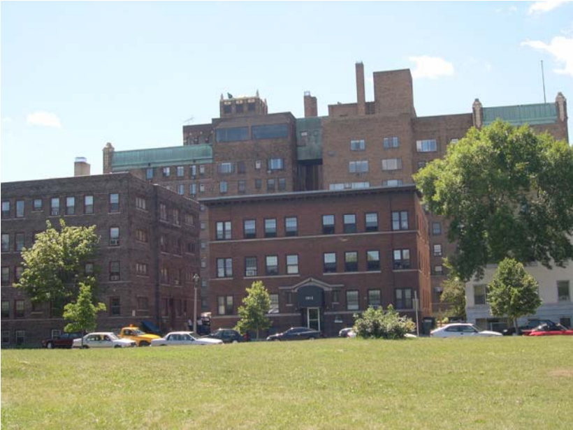
From center of site, towards Lafayette
