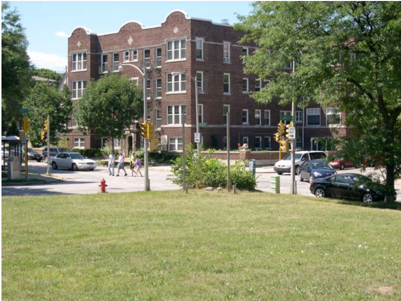
From center of site, towards corner Prospect and Lafayette
