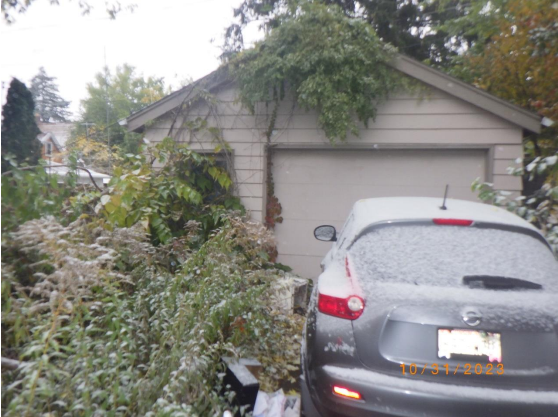
Initial Inspection-10/31/23 1716 East Iron Street
