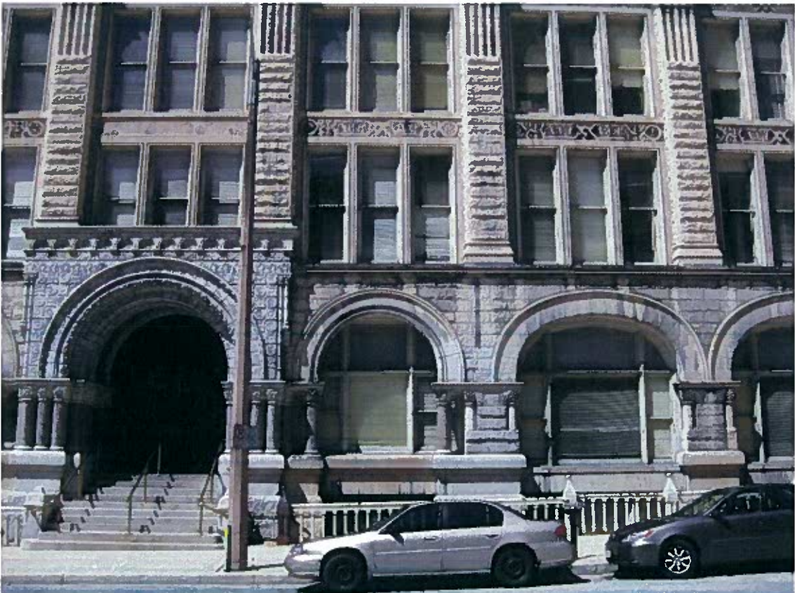
Photo 12: Broadway Façade entry detail
