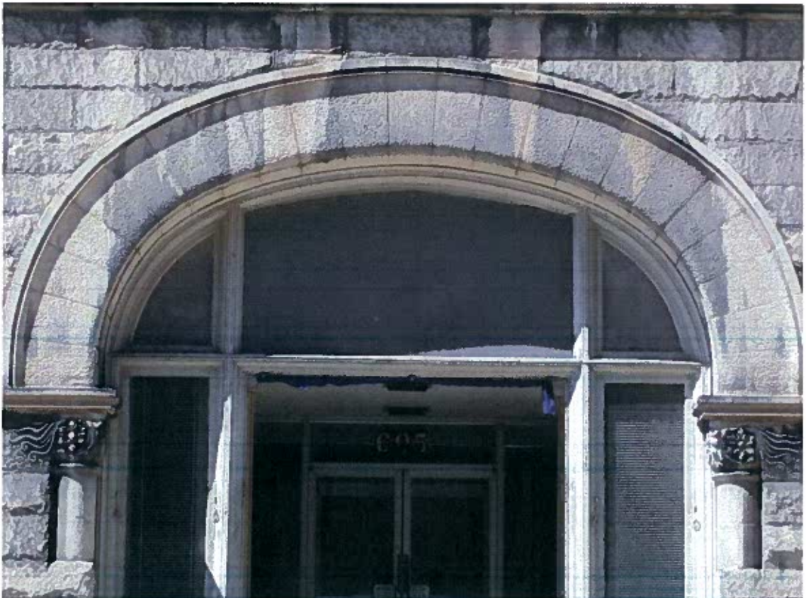
Photo 16: First Floor window detail
