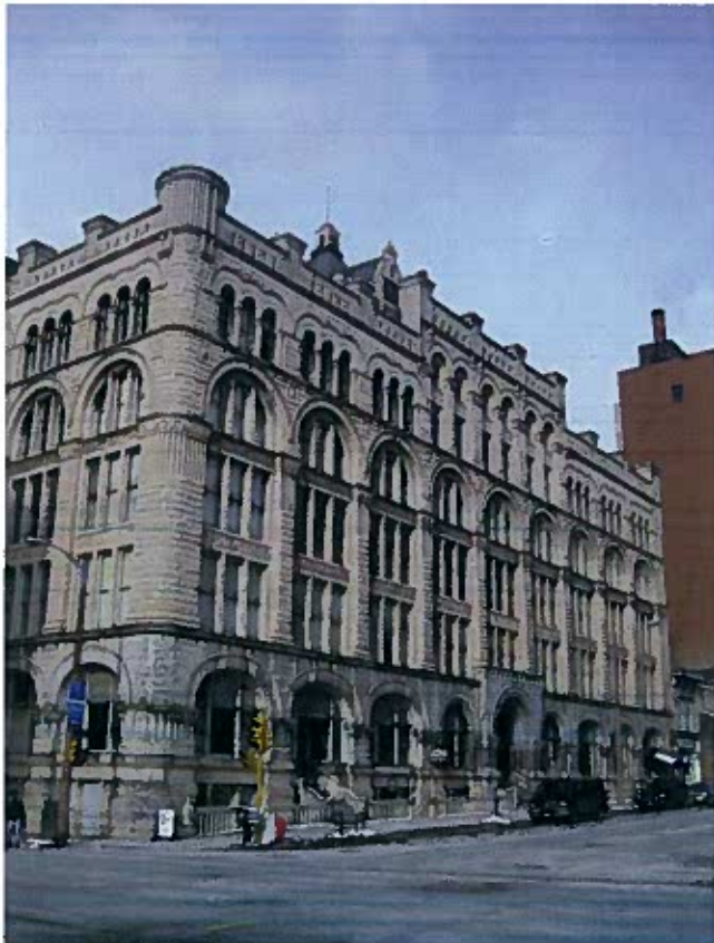
Photo 6: Broadway Façade looking Northwest
