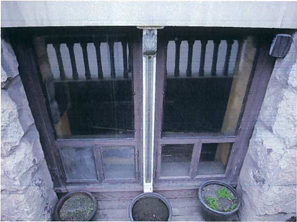
Photo 17: Ground Floor window detail
