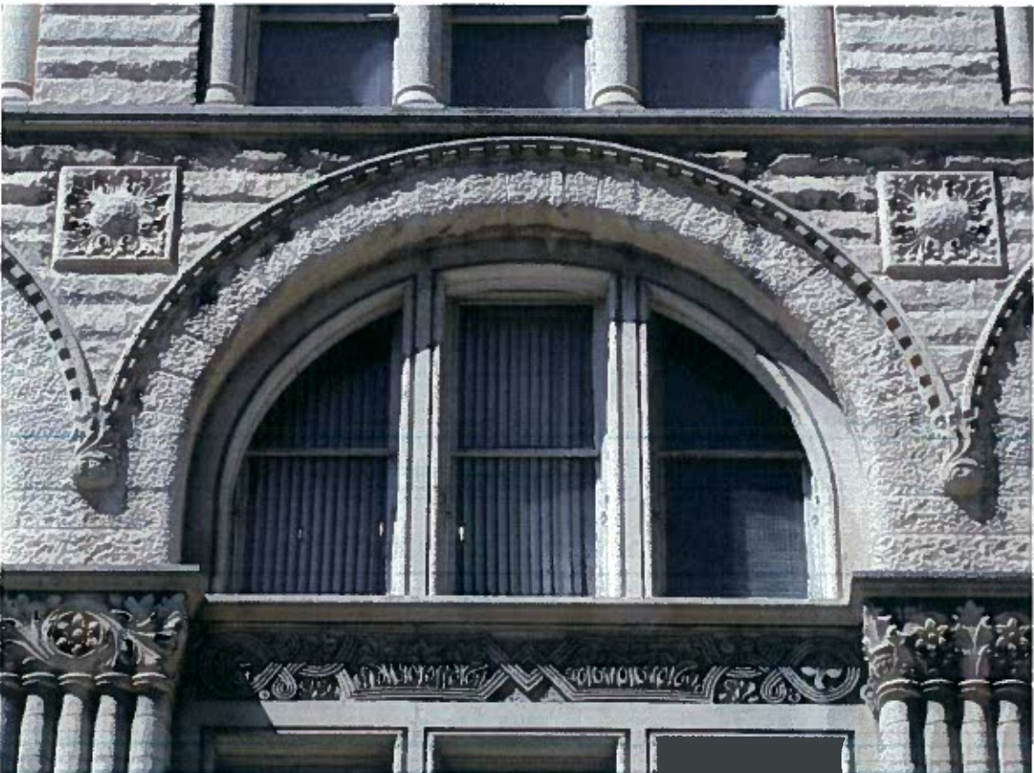
Photo 14: Fourth Floor window detail
