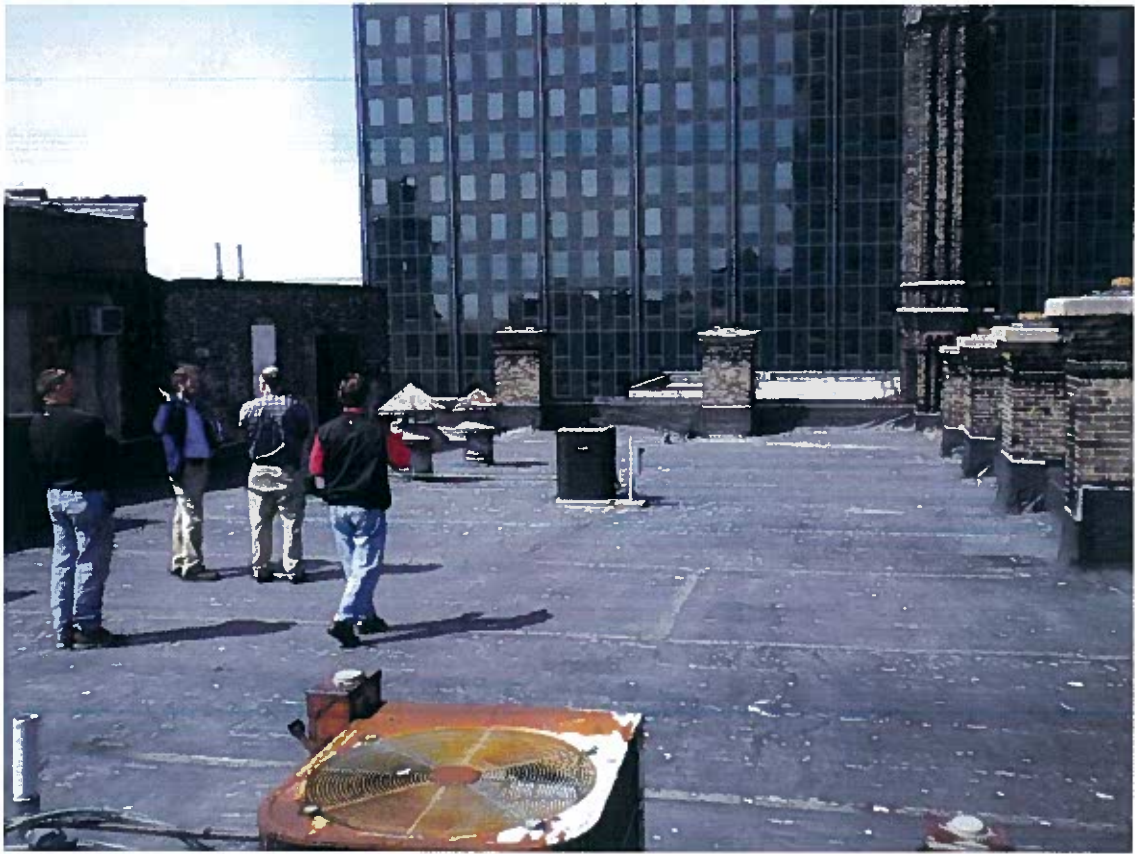
Photo 19: Roof, looking West
