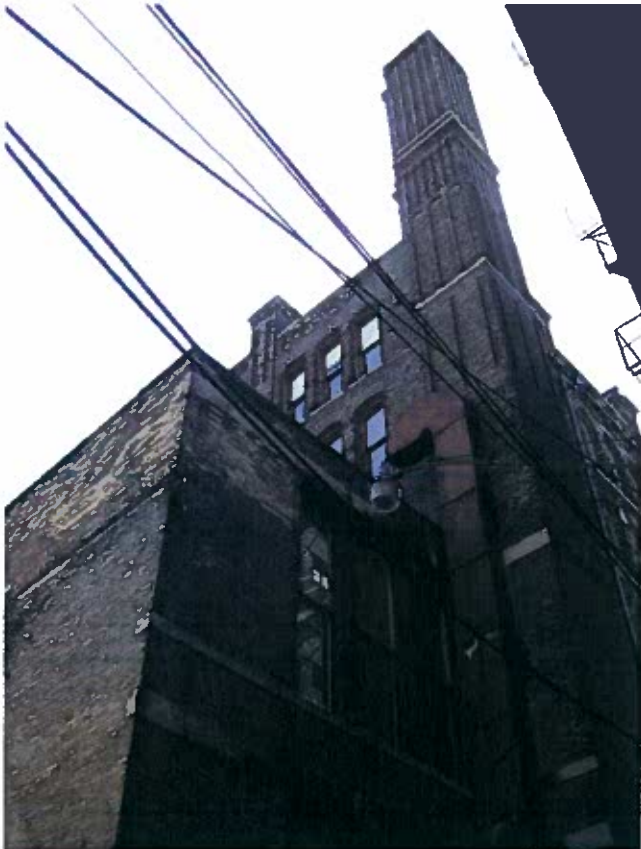
Photo 10: Alley Façade, looking South
