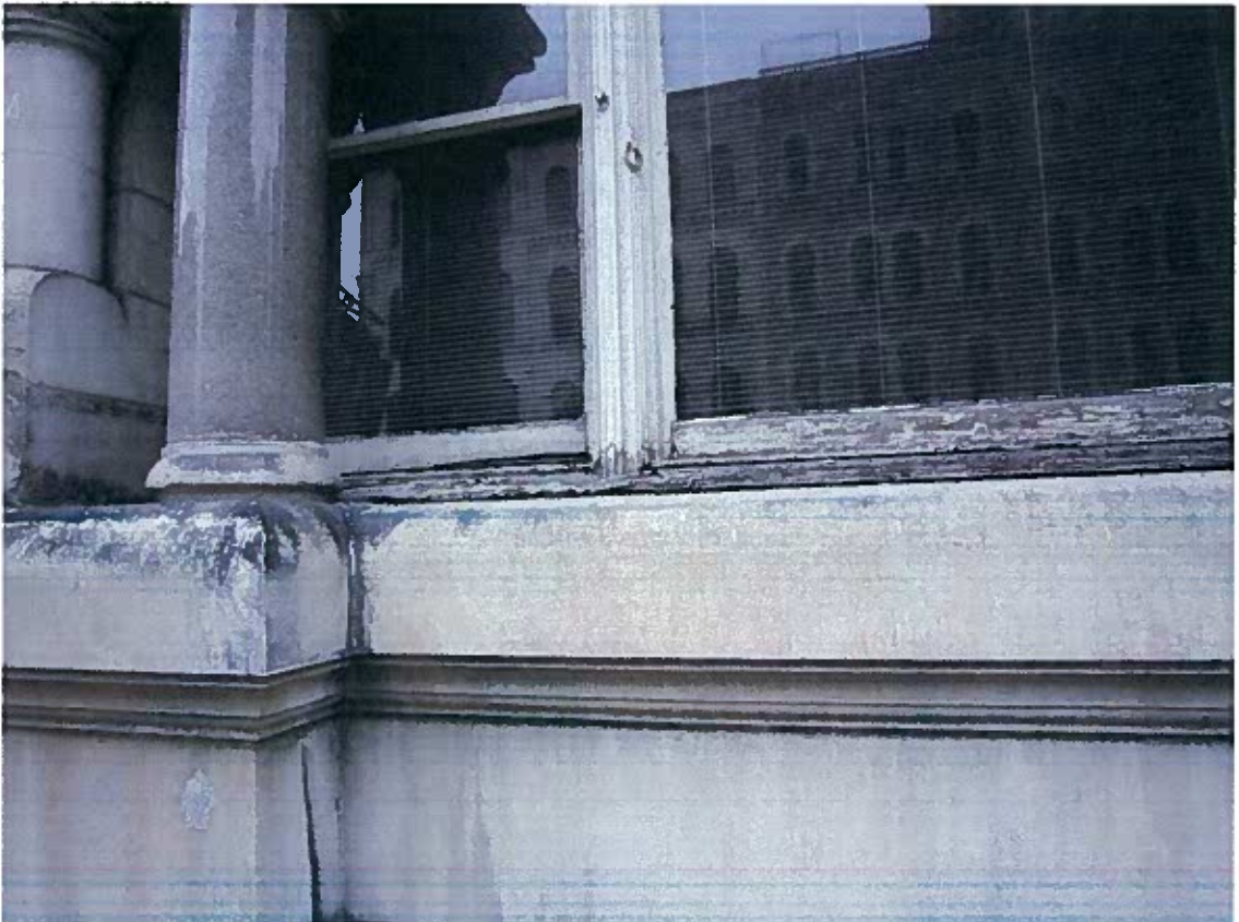
Photo 20: Typical window condition
