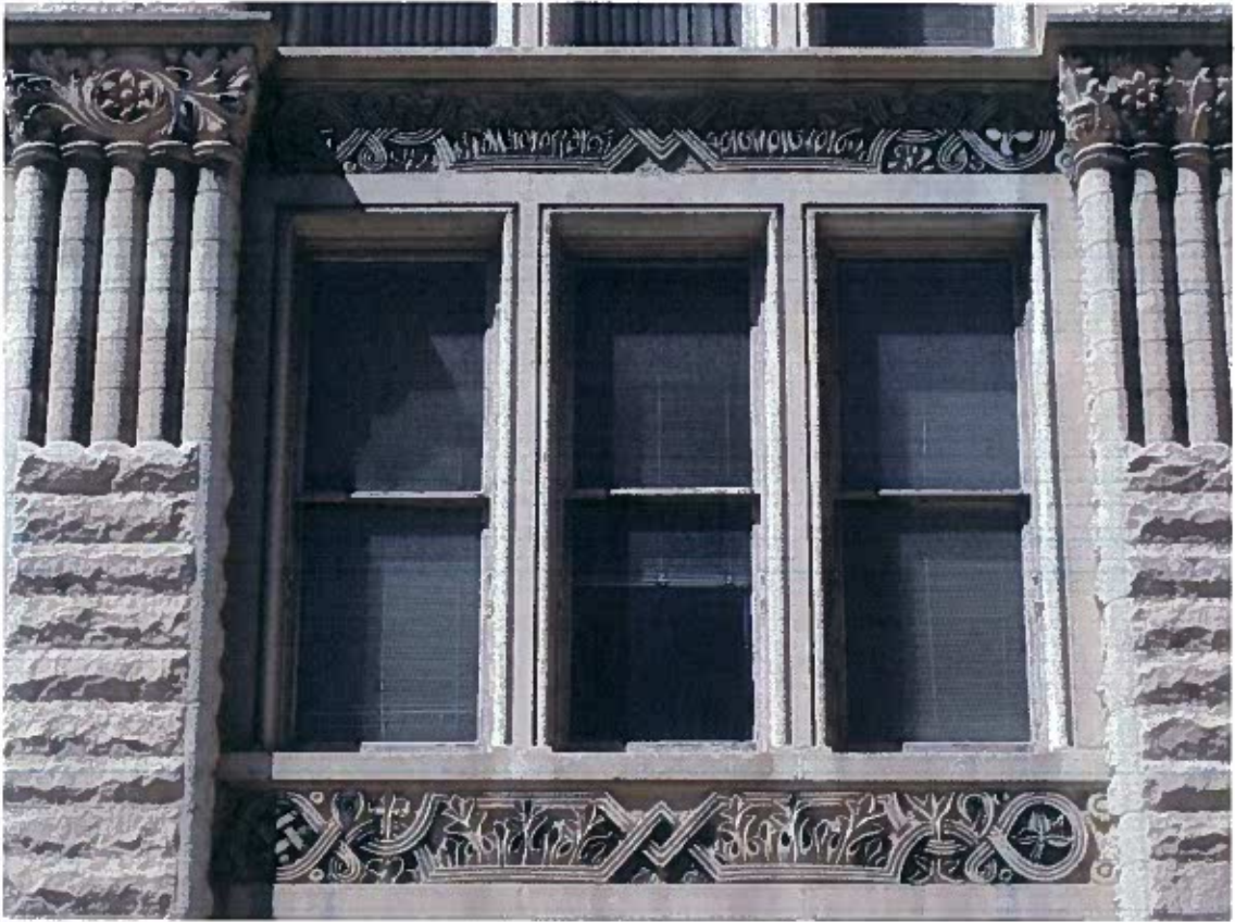
Photo 15: Third Floor window detail
