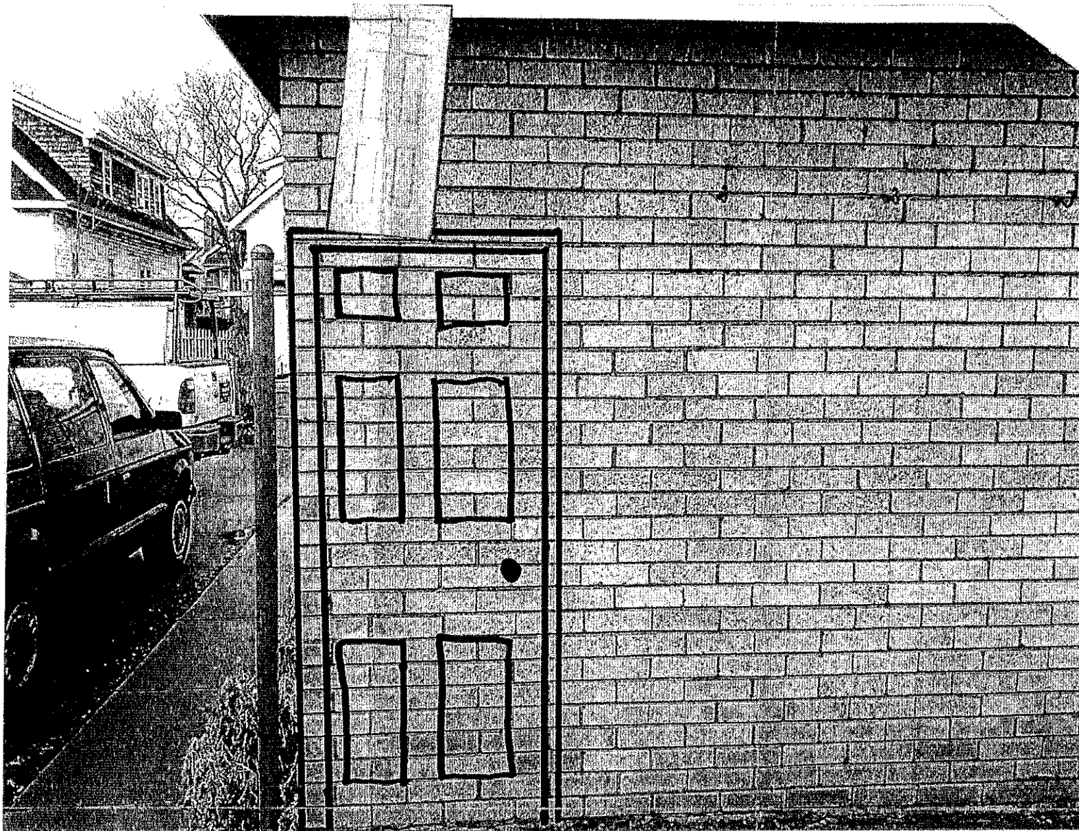
New service door to be installed in garage
