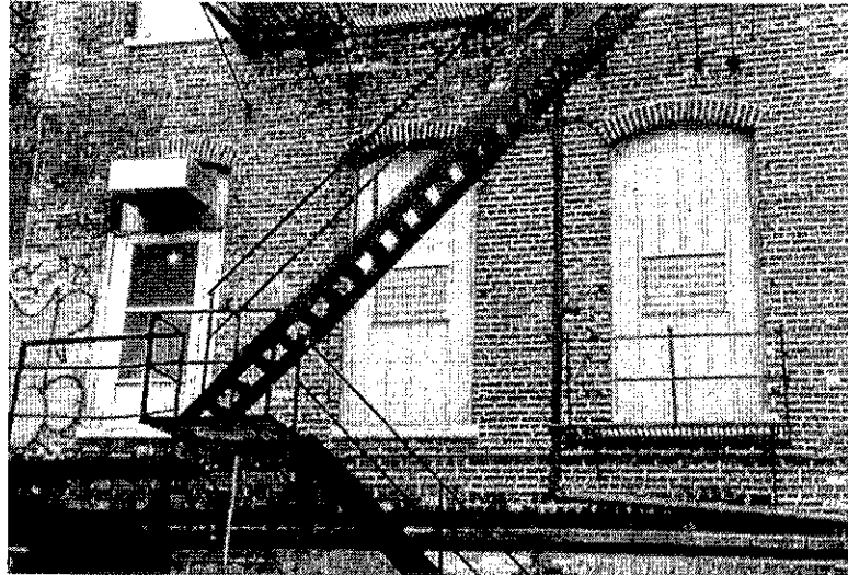
Two rear, alley facing windows to be replaced.
