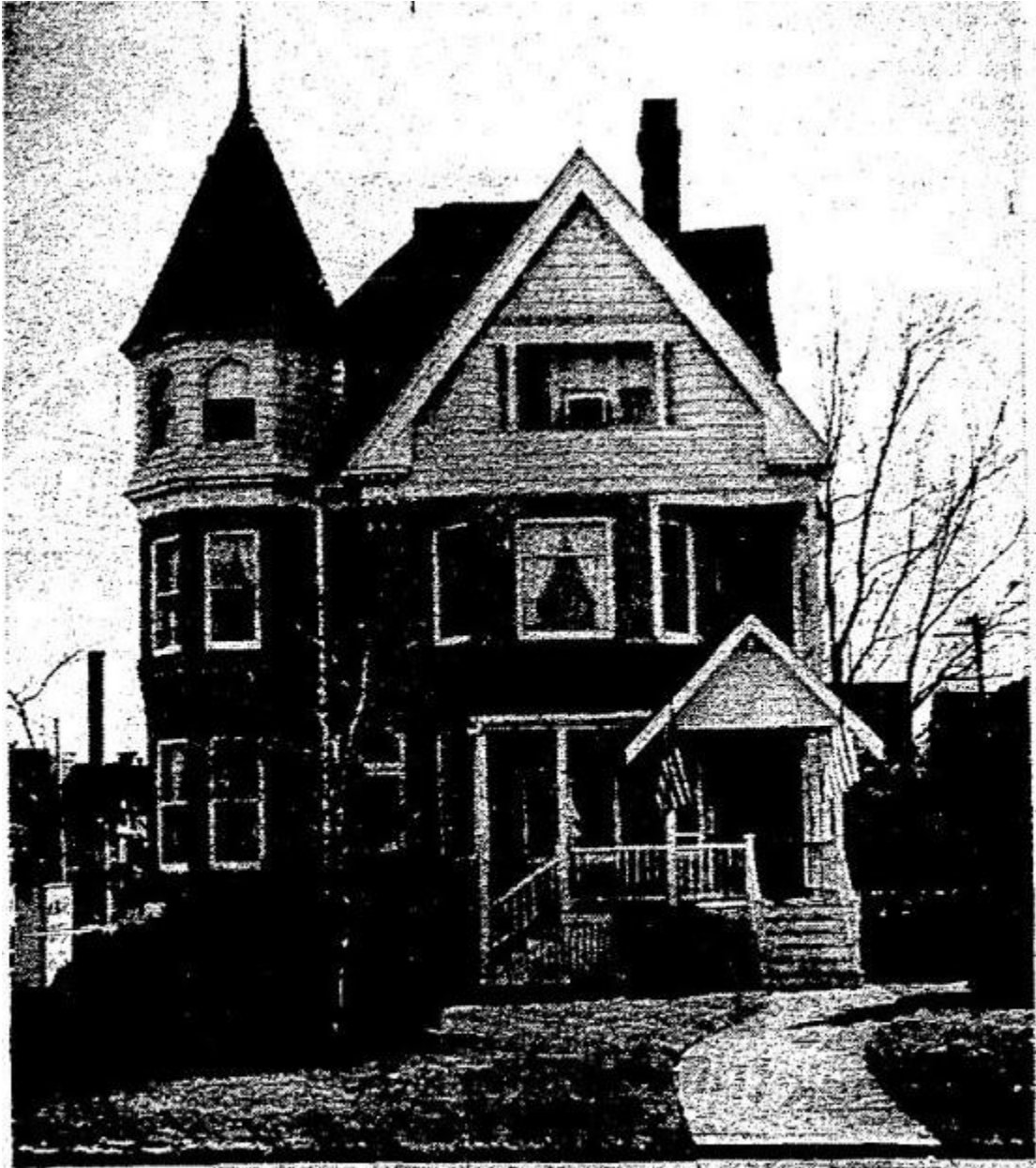
The exterior of the Realtors' building, a home built in 1892, has been restored to its turn of the century appearance. The original porch was duplicated; asphalt siding was replaced by cedar shake shingles on the third floor, the Cream City brick was cleaned and a new roof was added.
