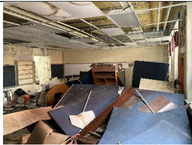
S239-S241-02: Interior View at far wall
