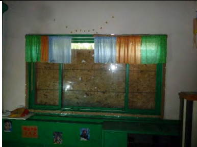
E113-01: Interior view
