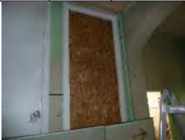
LC300-01: Interior view of window
