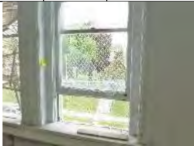
W311-01: Interior view of lower sash
