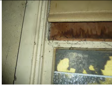
E104-02: Interior view of upper sash
