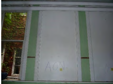
LC203-01: Interior view at center
