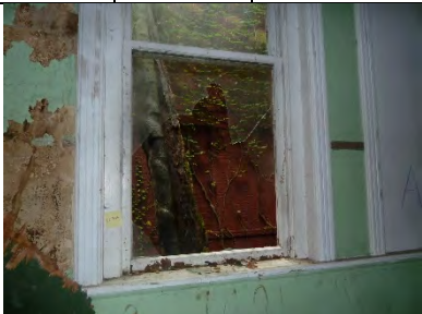
LC204-01: Interior view of lower sash
