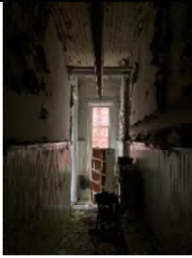
LC217-01: Interior view
