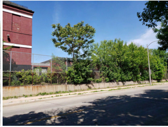
East Elevation of one story addition. (Largely obscured by vegetation.) Tags are E106-E113
