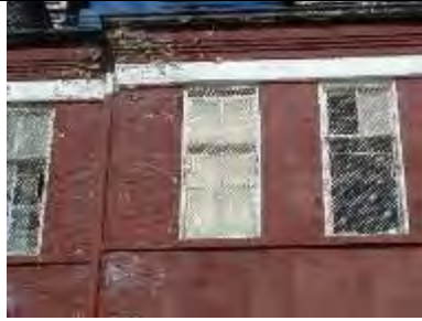
S322-02: Exterior view of window at center
