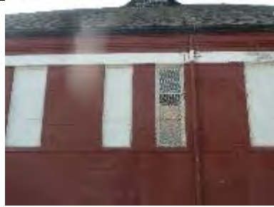
N306-02: Exterior view on left
