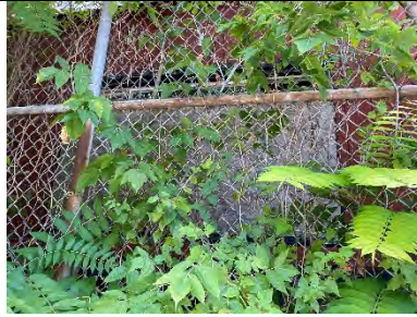
E112-02: Exterior view
