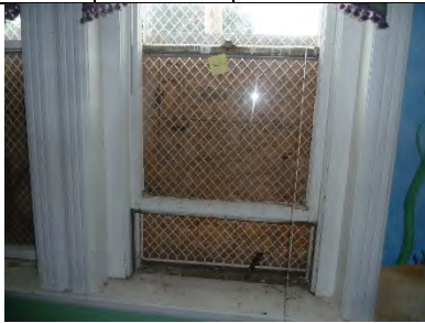
W203-01: Interior view of lower sash
