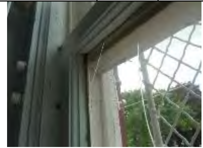
W310-03: Blown corner of upper sash
