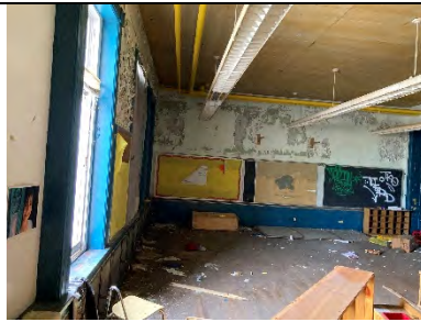
E207-E209-02: Interior View at far wall
