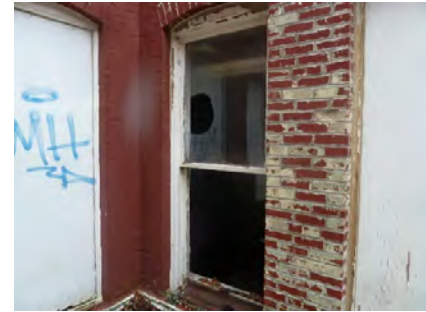
LC205-04: Exterior view
