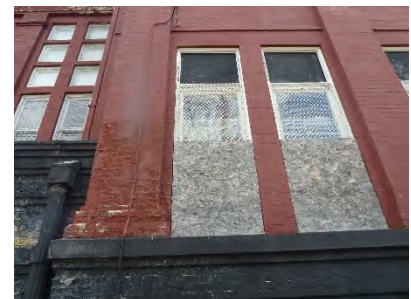
W203-04: Exterior view on left
