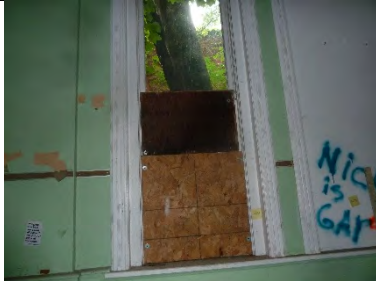
LC223-01: Interior view of lower sash
