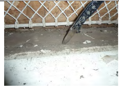
W203-03: Exterior jamb condition
