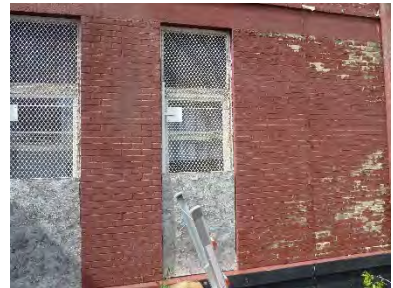
N245-04: Exterior view at right
