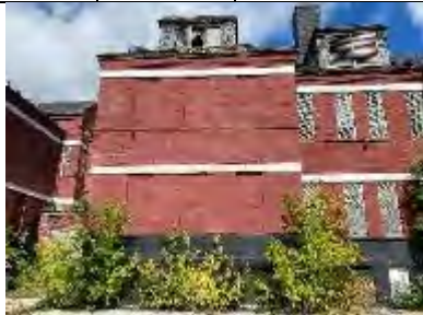
S338-S340-01: Exterior view
