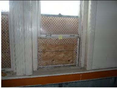
W211-01: Interior view of lower sash
