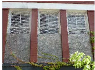
S238-04: Exterior view at right
