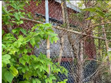
E113-02: Exterior view
