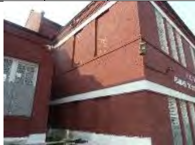
N319-N321-01: Exterior view of bricked-in openings
