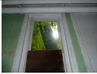
LC223-02: Interior view of upper sash
