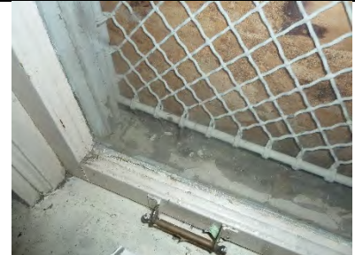
W212-03: Exterior jamb condition
