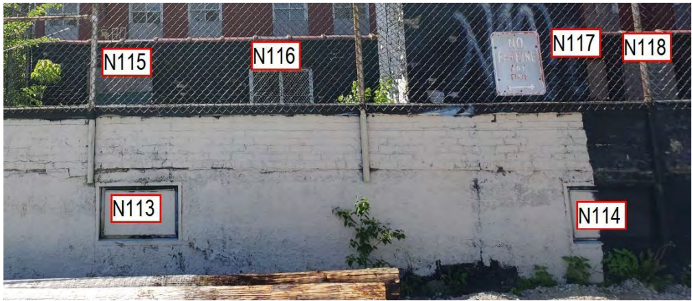
North Elevation - Lower Center Section
