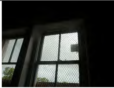
N217-02: Interior view of upper sash
