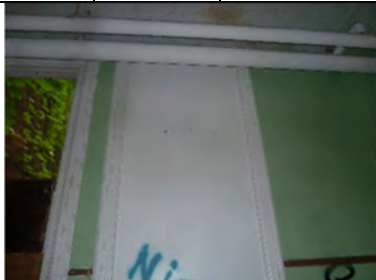
LC222-01: Interior view
