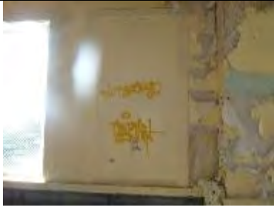
S322-01: Interior view of window
