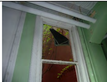
LC200-02: Interior view of upper sash
