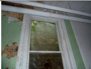
LC204-02: Interior view of upper sash
