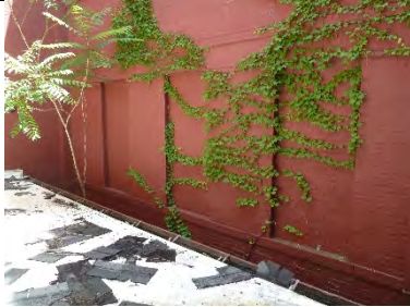
LC213-LC215-01: Exterior view (l to r)
