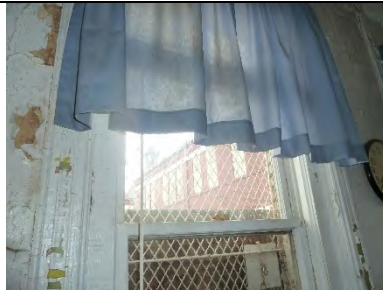
N245-02: Interior view of upper sash
