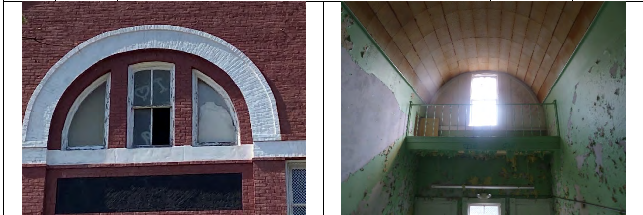
E400/E401/E402-01: Exterior view from left
