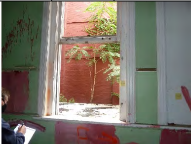
LC209-01: Interior view of lower sash
