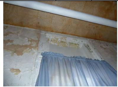
N245-03: View of fixed transom head
