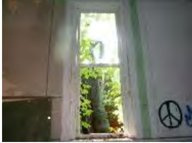
LC323-01: Interior view of window
