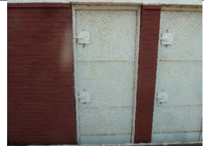
N200-03: Exterior view at center
