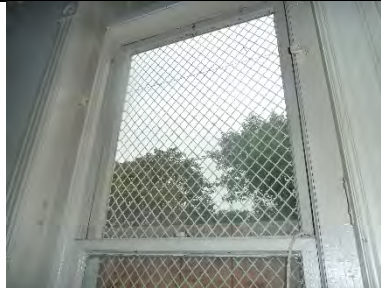
W212-02: Interior view of upper sash
