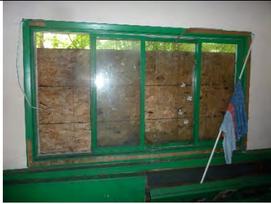
E112-01: Interior view
