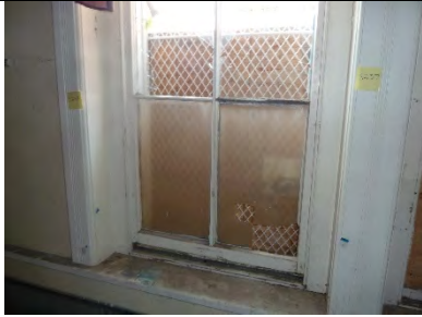
S238-01: Interior view of lower sash
