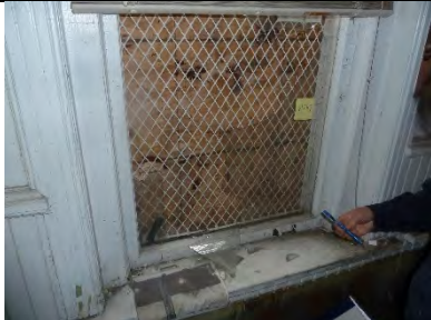
N242-01: Interior view of lower sash
