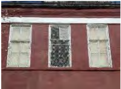
S323-04: Exterior view at center
