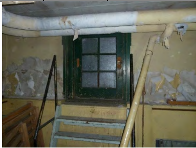
E105-01: Interior view of exit door
