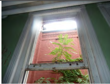
LC209-02: Interior view of upper sash
