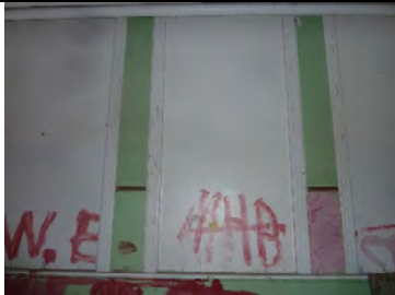
LC207-01: Interior view at center
