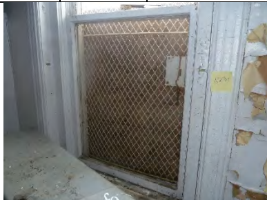
N231-01: Interior view of lower sash
