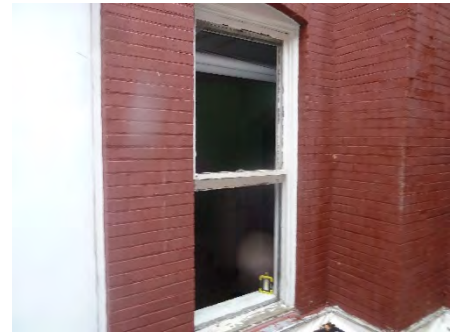
LC209-04: Exterior view
