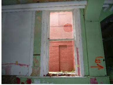
LC205-01: Interior view
