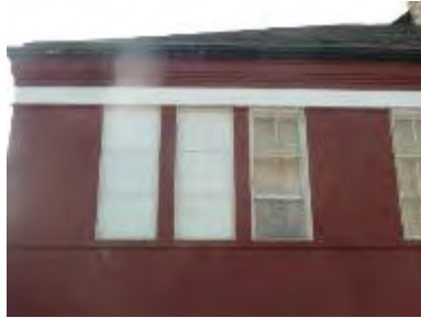
N301-02: Exterior view at center
