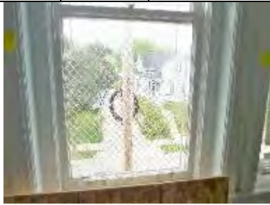
W310-01: Interior view of lower sash
