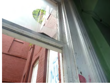
LC205-02: Interior view meeting rail
