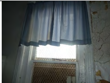
N231-02: Interior view of upper sash
