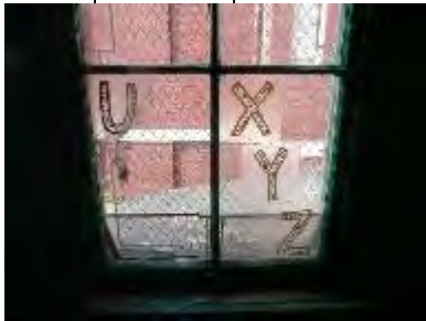
S332-01: Interior view of lower sash
