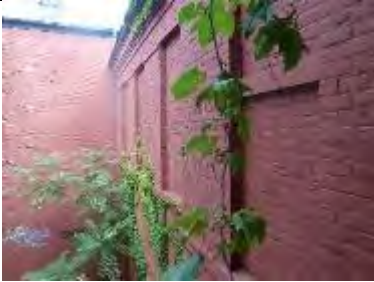
LC313-LC316-01: Exterior view (l to r)
