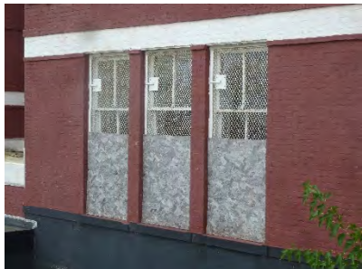
N218-04: Exterior view at center
