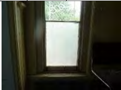
E310-01: Interior view of lower sash
