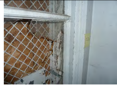
S226-03: Screw repair at sash corner
