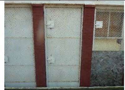
N201-03: Exterior view at center
