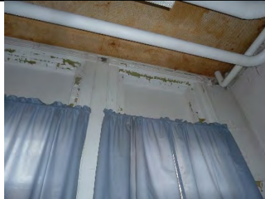
N242-02: Interior view of upper sash
