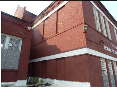
N214-N216-01: Exterior View at lower center
