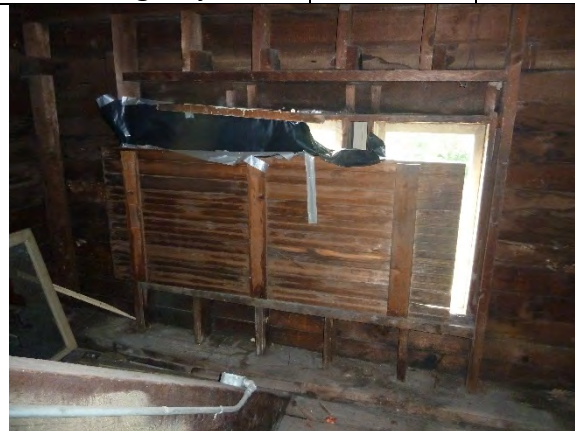
S404/S405/S406-01: Interior view from right
