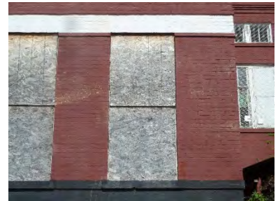
S226-04: Exterior view at center
