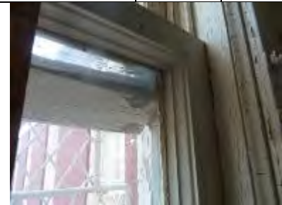
N334-03: Blown corner of upper sash
