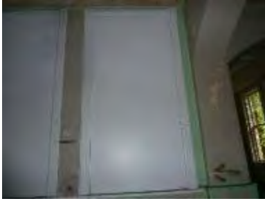
LC305-01: Interior view
