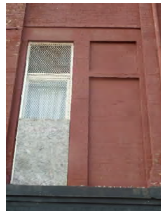
N231-04: Exterior view on left
