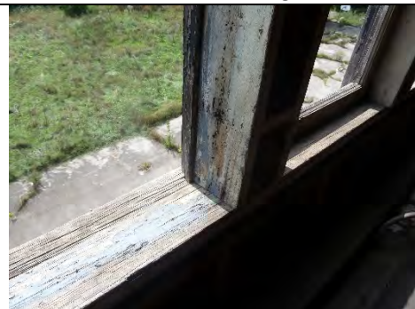
S413/S414/S415-03: Interior view of jamb
