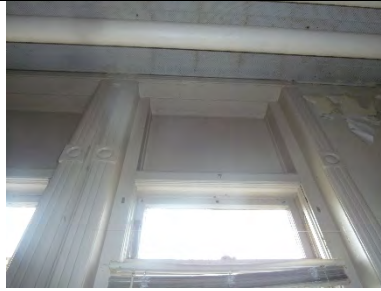
W211-02: Interior view of upper sash
