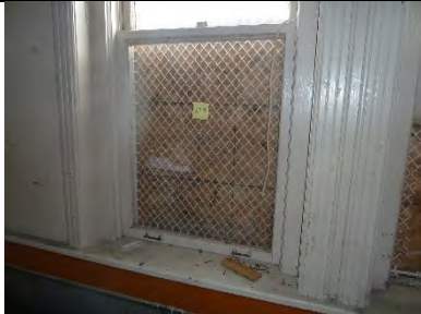
W212-01: Interior view of lower sash
