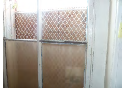
S238-03: Screw repair at sash corner
