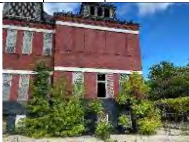
S345-S347-01: Exterior view
