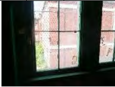
S337-01: Interior view of lower sash
