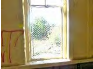
S323-01: Interior view of lower sash
