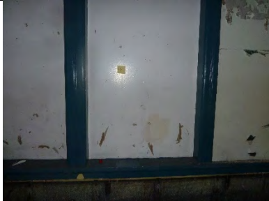
N200-01: Interior view of lower sash
