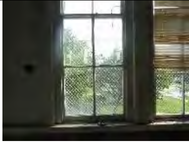
E305-01: Interior view of lower sash
