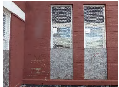
N241-04: Exterior view on left
