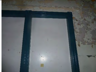
N200-02: Interior view of upper sash
