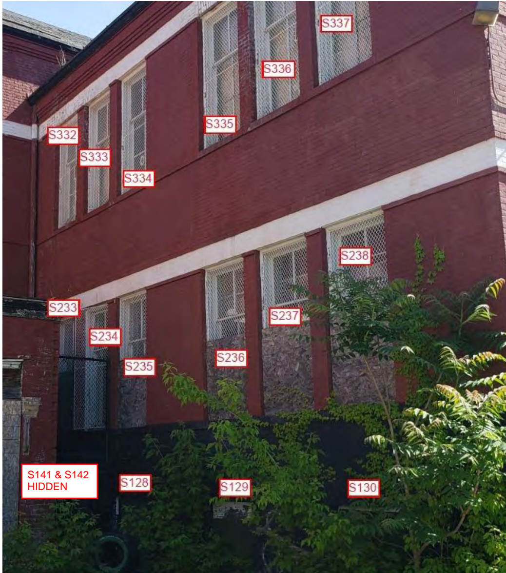
South Elevation - Courtyard (east elevation wall of courtyard)
