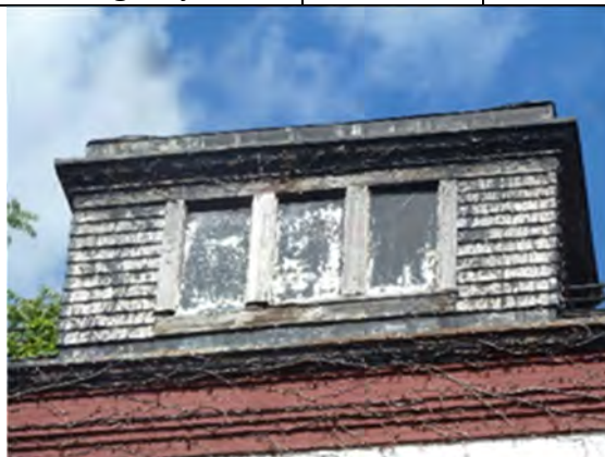
S400/S401/S402-01: Exterior view from left
