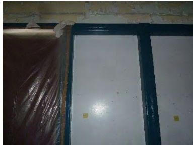
N201-02: Interior view of upper sash
