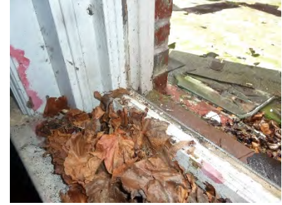
LC205-03: Bottom of sash is split out
