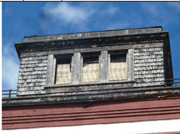
S404/S405/S406-01: Exterior view from left
