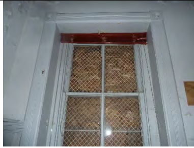
S226-02: Interior view of upper sash
