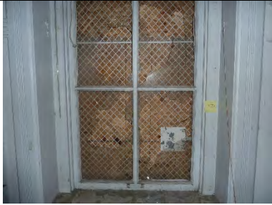
S226-01: Interior view of lower sash
