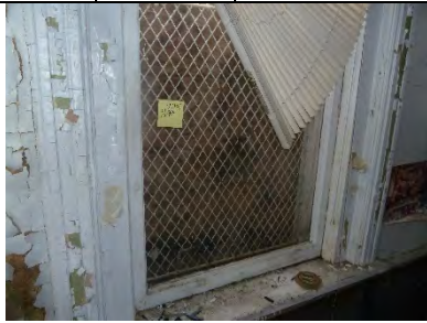
N245-01: Interior view of lower sash
