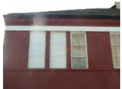
N302-04: Exterior view on right
