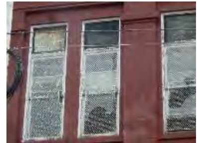
W310-03: Blown corner of upper sash
